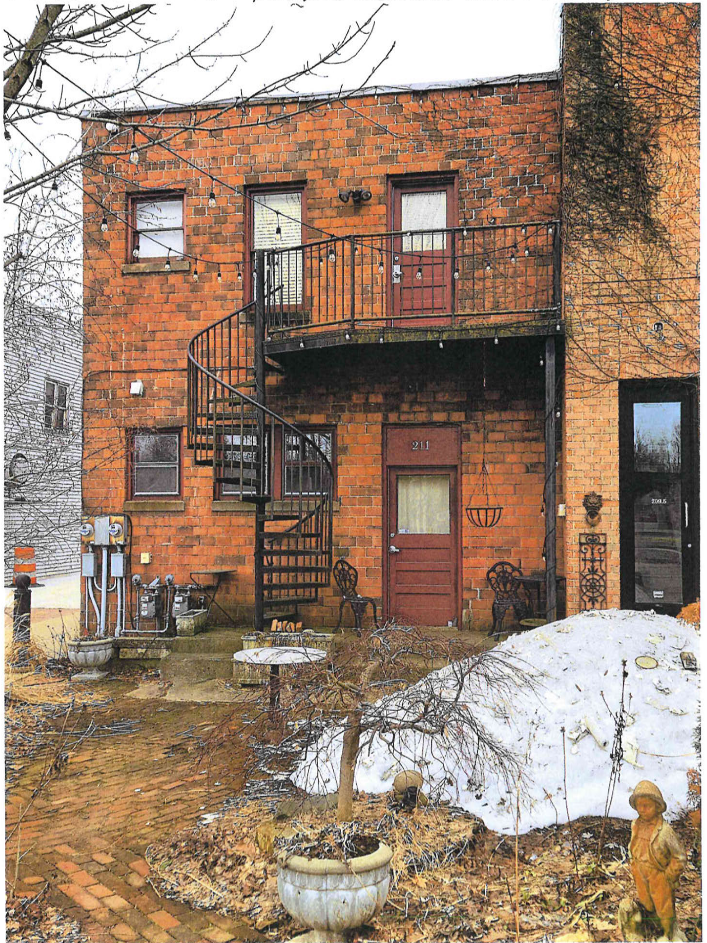
611 E. FRONT ST. - REAR FACADE EXISTING
