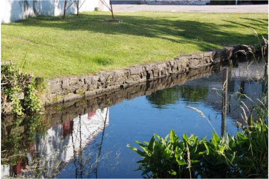
The Buchanan Preservation Society asks that the City rebuild both the collapsed and the deteriorated portions of the northerly mill race wall; and since the race is a contributing resource to the Downton Historic District and an integral component of Pears Mill operations, the Society also asks to be a partner in the design and execution of this work.
