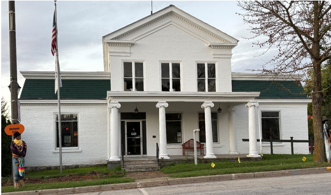
View looking south from W Front Street.
