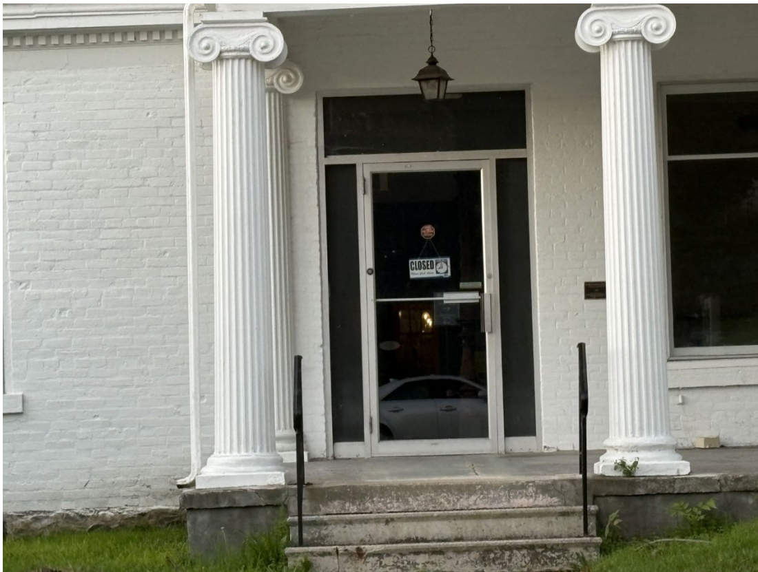
View looking south from W Front Street of existing front door proposed to be replaced.
