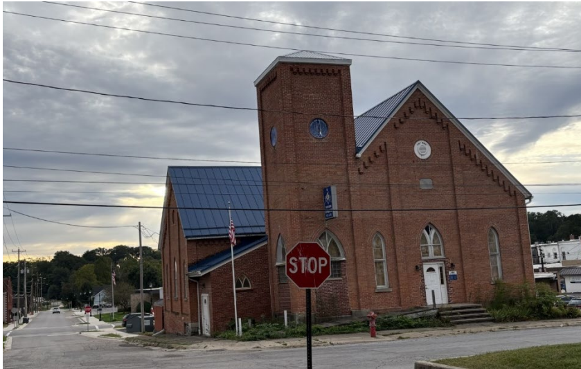
New roof view from W Dewey Street
