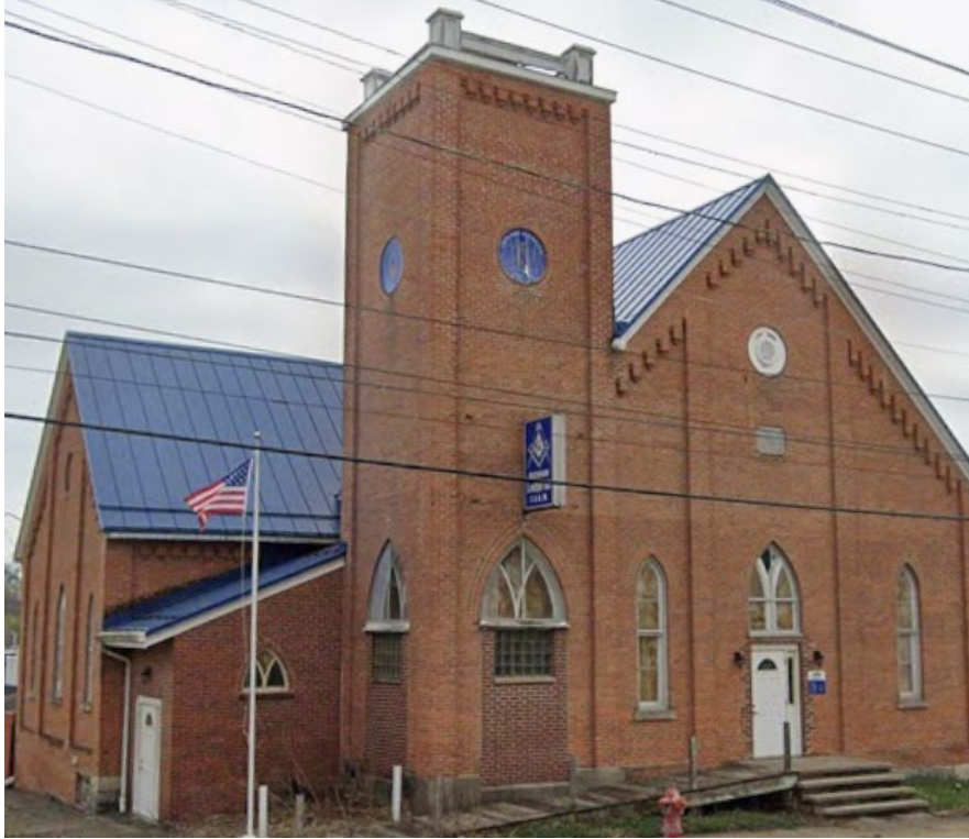
Old roof view from W Dewey St. Google Street View April 2026
