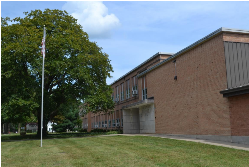
Moccasin School, 416 Moccasin St. (located in North-West District, c. 1950)**
