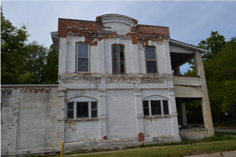
Zinc Collar Pad Building, 304 S. Oak (2009)
