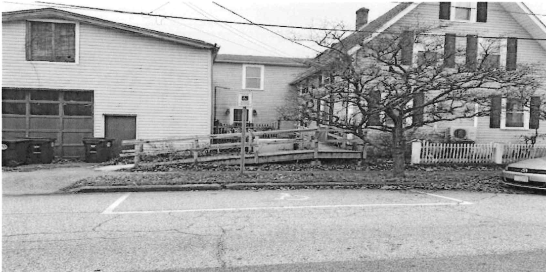
Accessible parking space on First Street adjacent to 204 State Street
