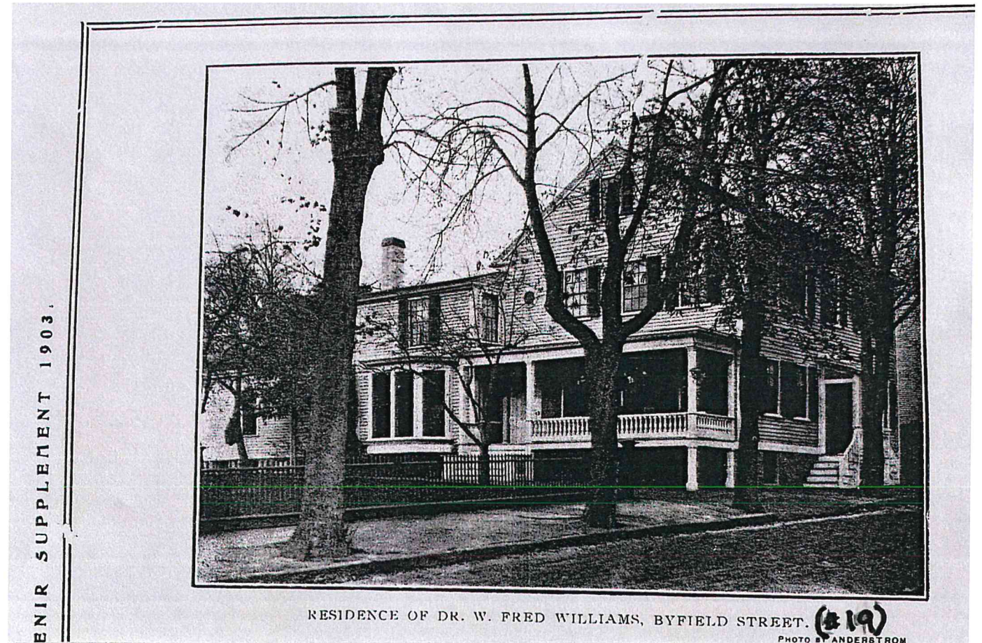
Photo #4: 1903 Photograph of Historic Addition
