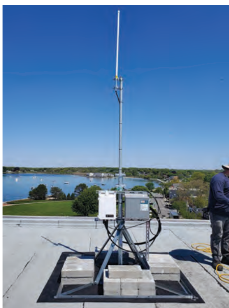
Antennae for new smart meter system.
