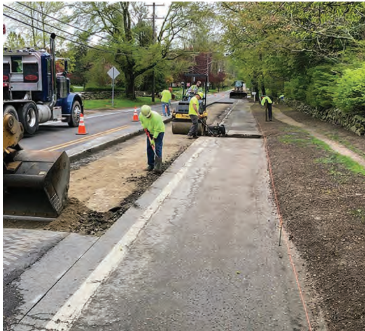
Paving the road after water main installation.
