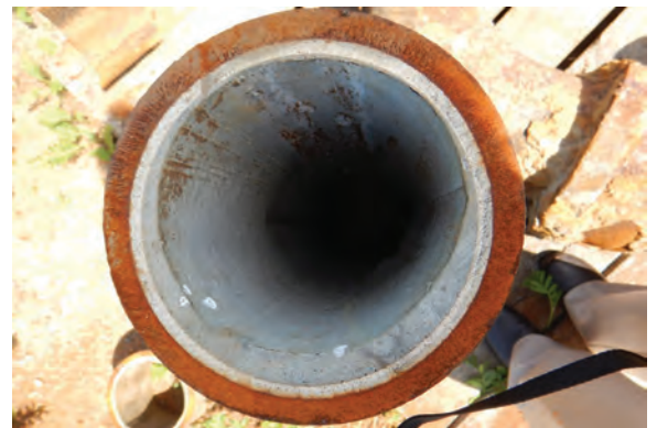
Old cast iron pipe with new cement lining.
