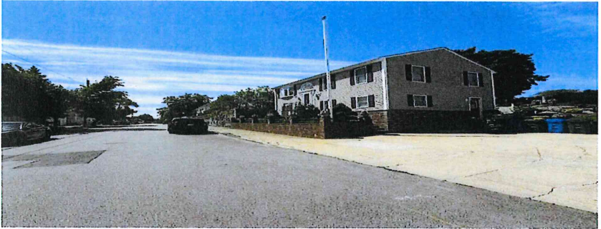
19 Second School Street- south view
