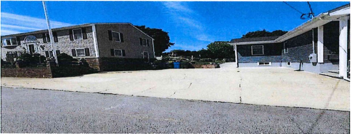
19 Second School Street-West view of shared driveway between 19 Second School Street and 27 Second School Street. Property line shows that 19 School Street has one off-street parking space.
