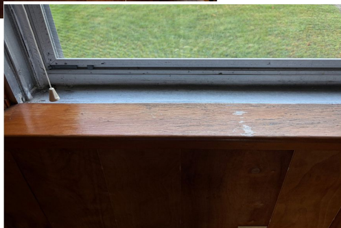
Window #4 Back Porch interior
