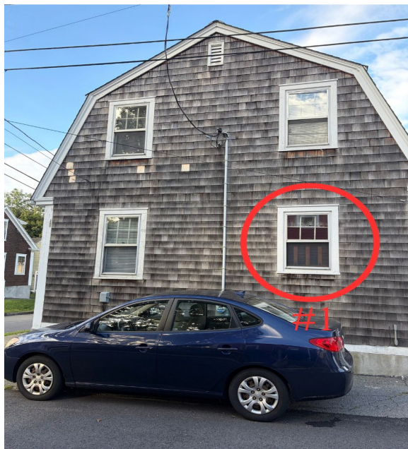
Window #1 Kitchen Exterior
