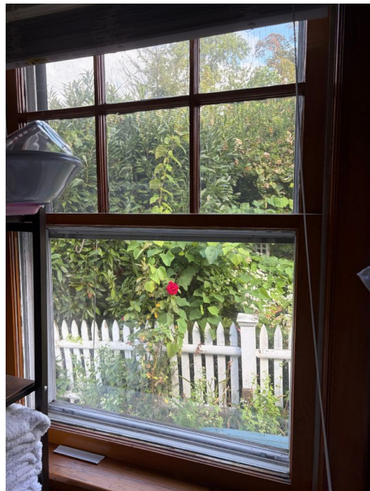
Window #3 Back Porch interior
