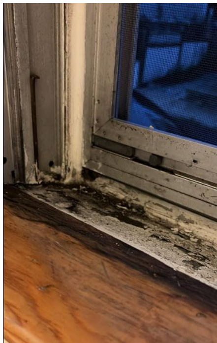
Window #1 Kitchen interior
