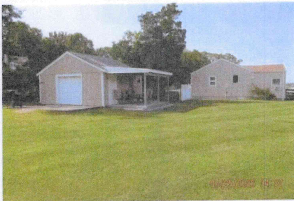
Cottage & Garage - to be demolished
