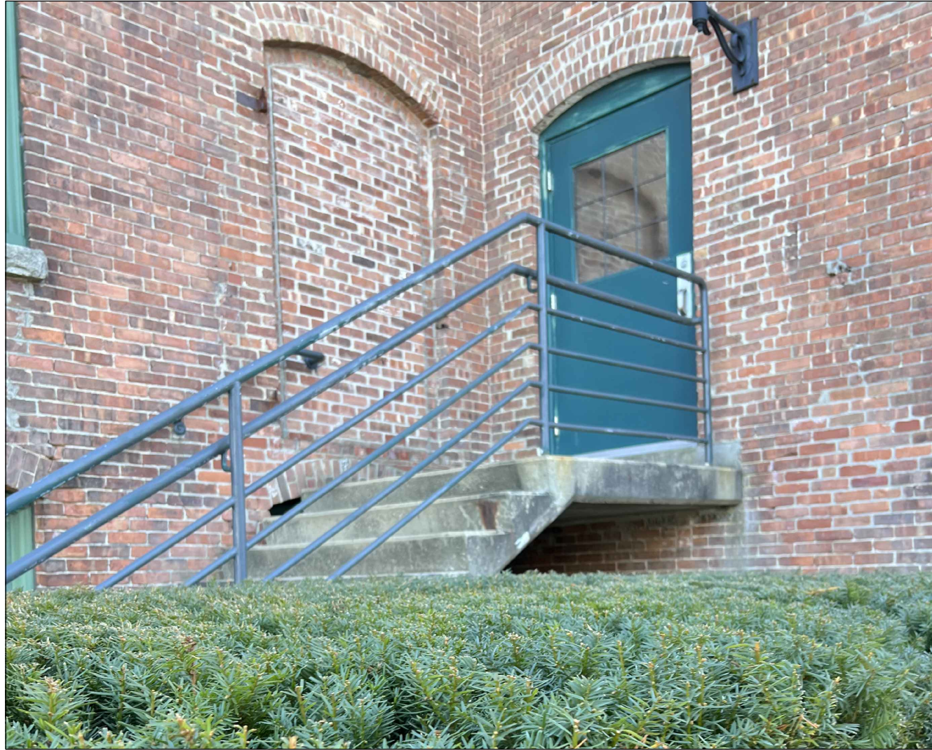
2 EXISTING STAIR AND RAILING
