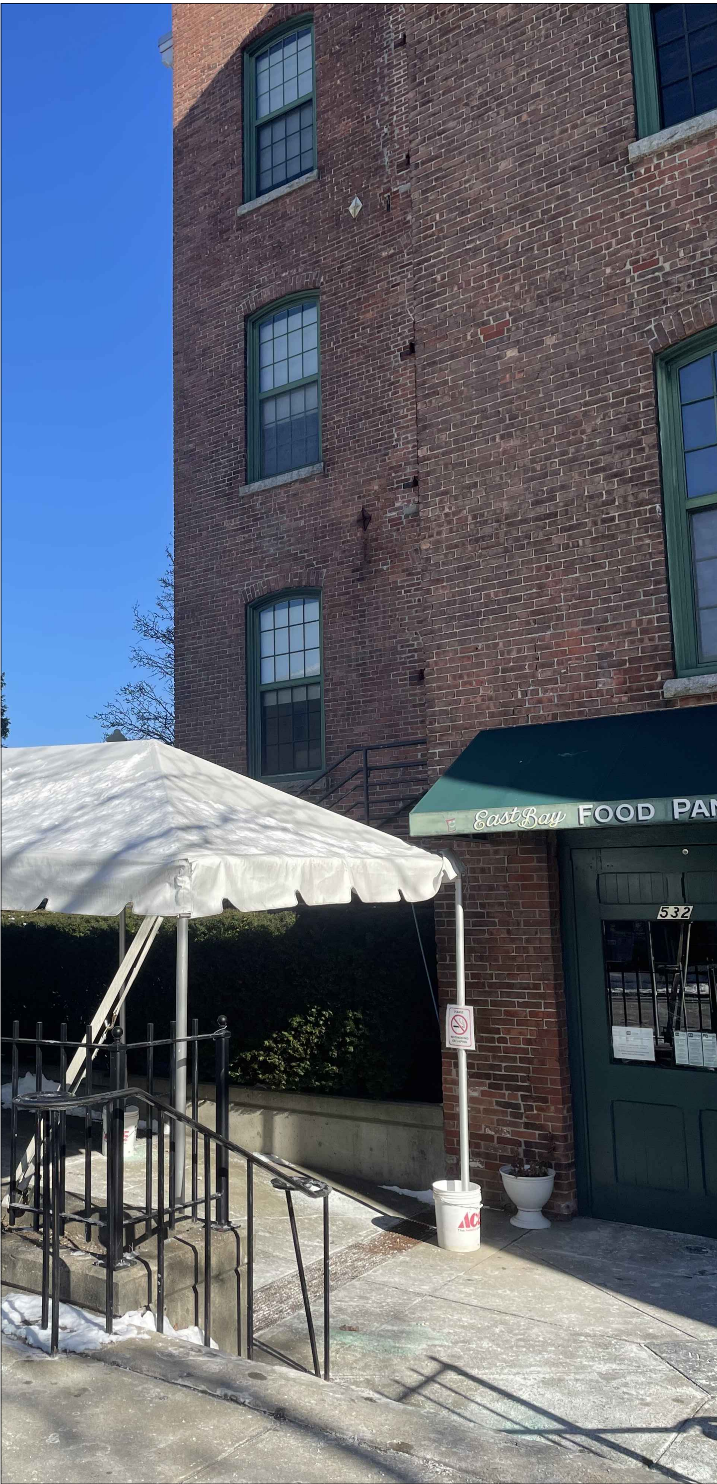
4 WEST ELEVATION PHOTOGRAPH
