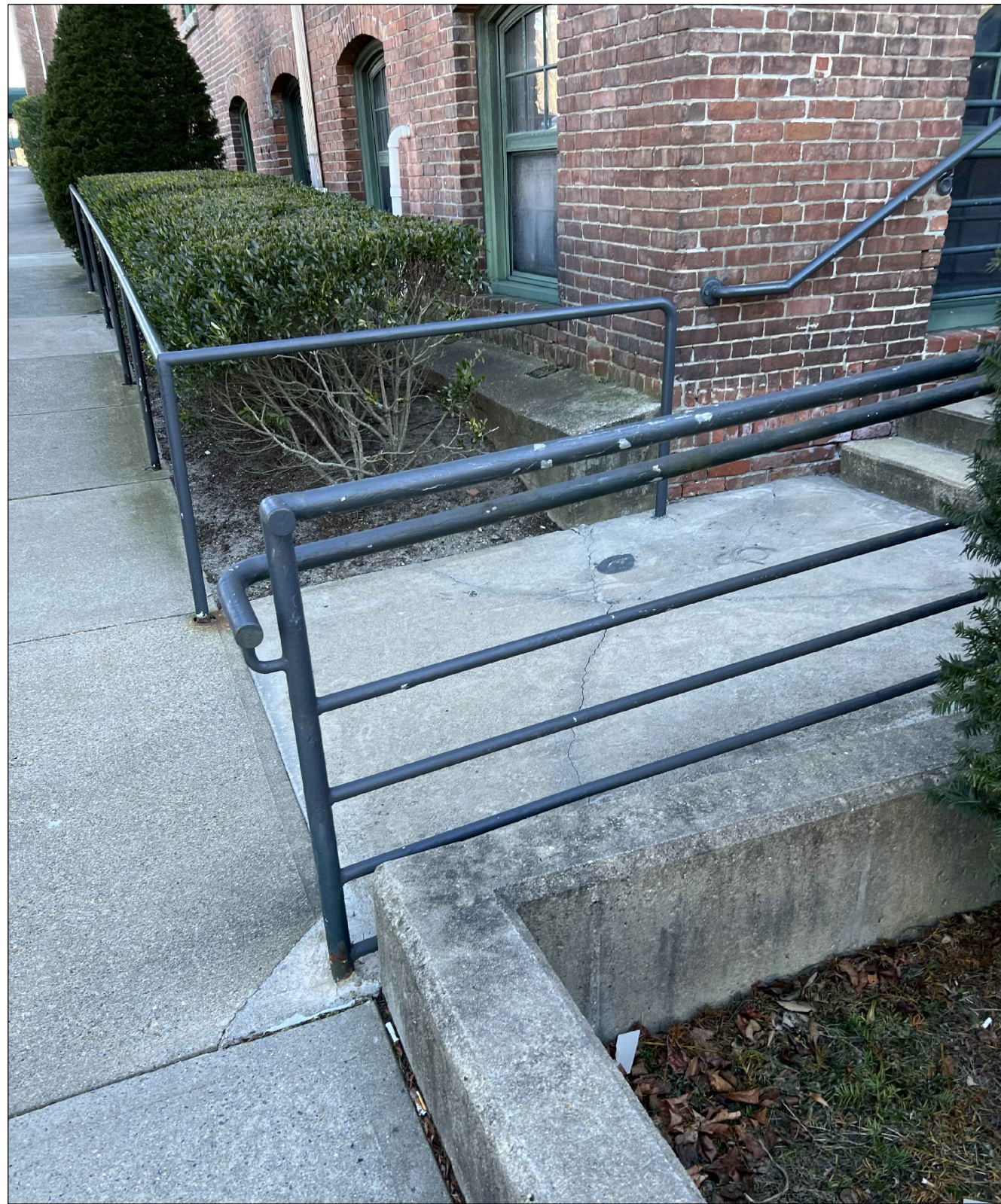
3 EXISTING RAILING EXAMPLE
