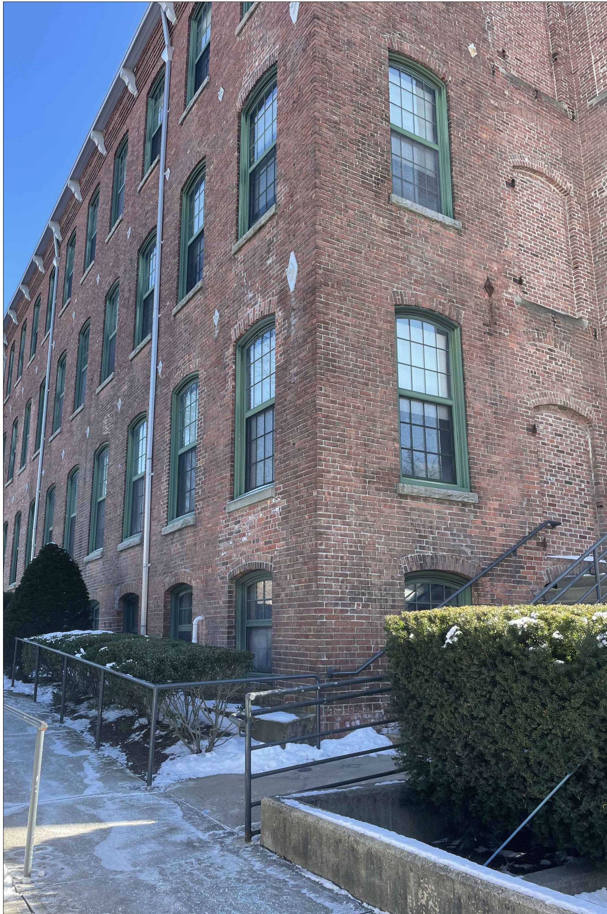
1 NORTHWEST ELEVATION PHOTOGRAPH
