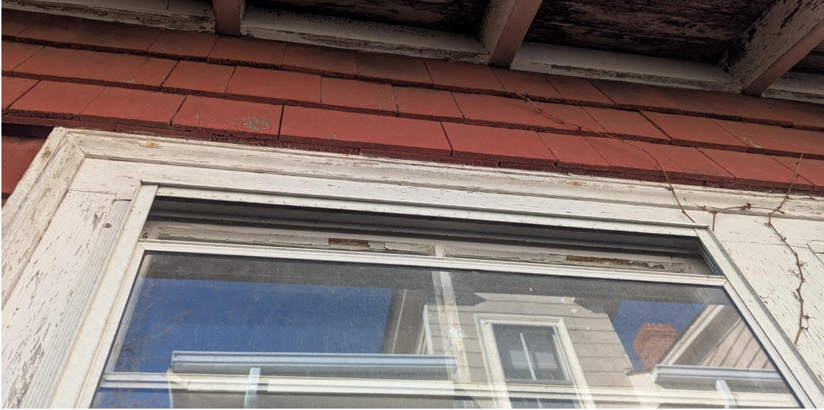
Cracked/missing glazing compound
