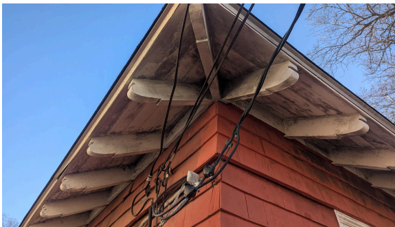
Exposed Rafter Tails & Tripled Shingles over window
