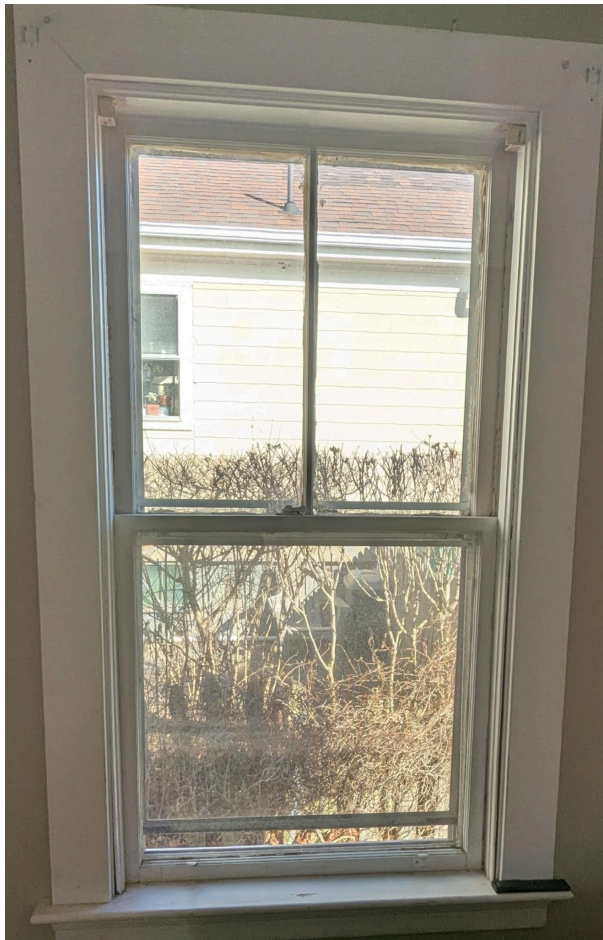
2-over-1 window (east elevation)
