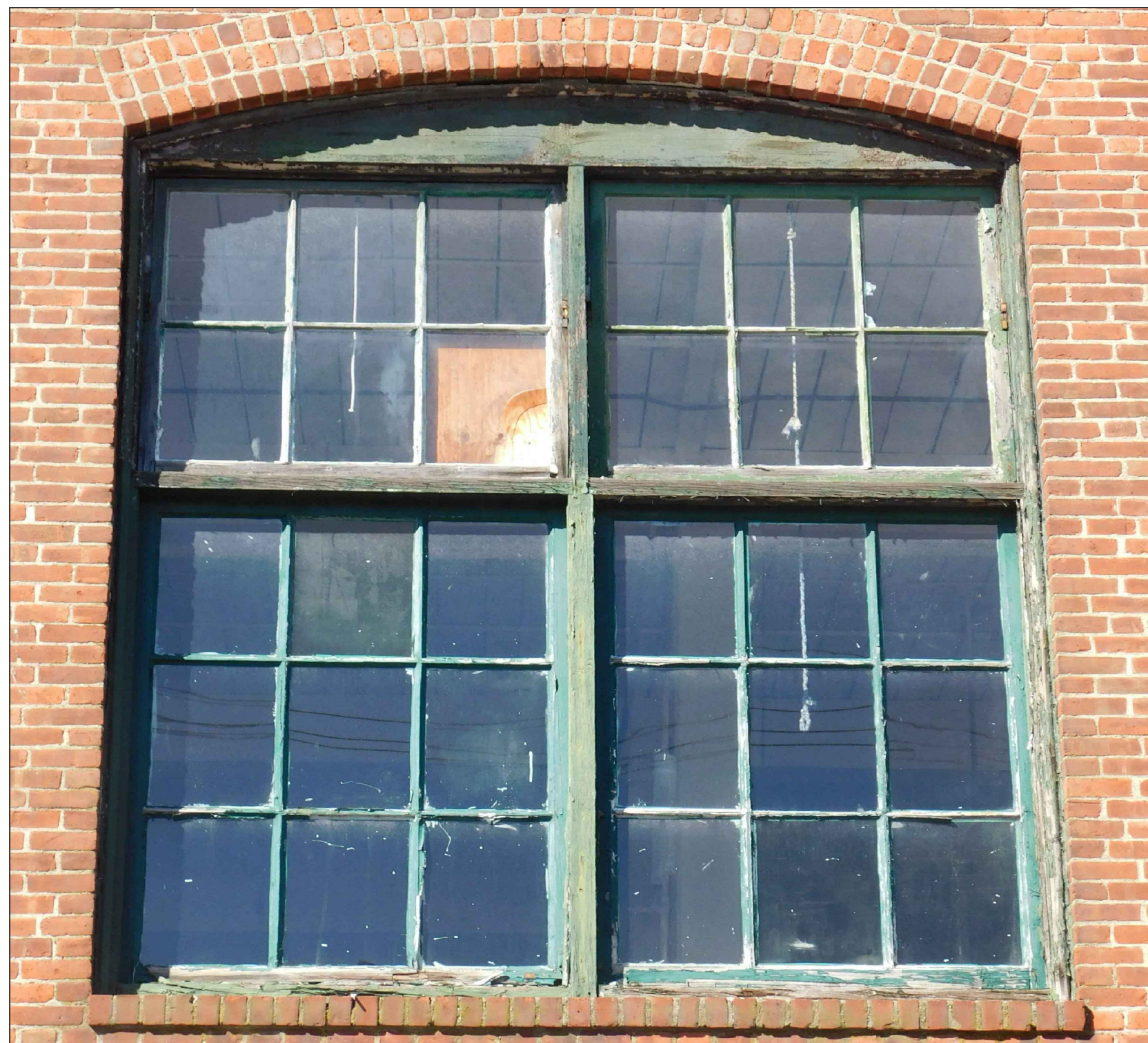
Building 7 Original Wooden Window Exterior
