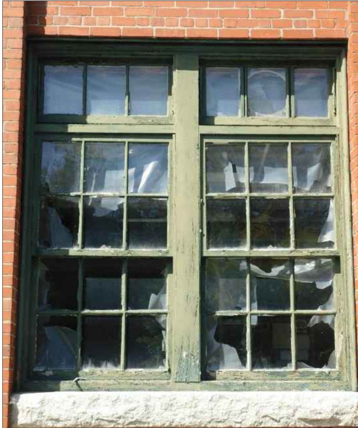
Building 4 Original Wooden Window Exterior
