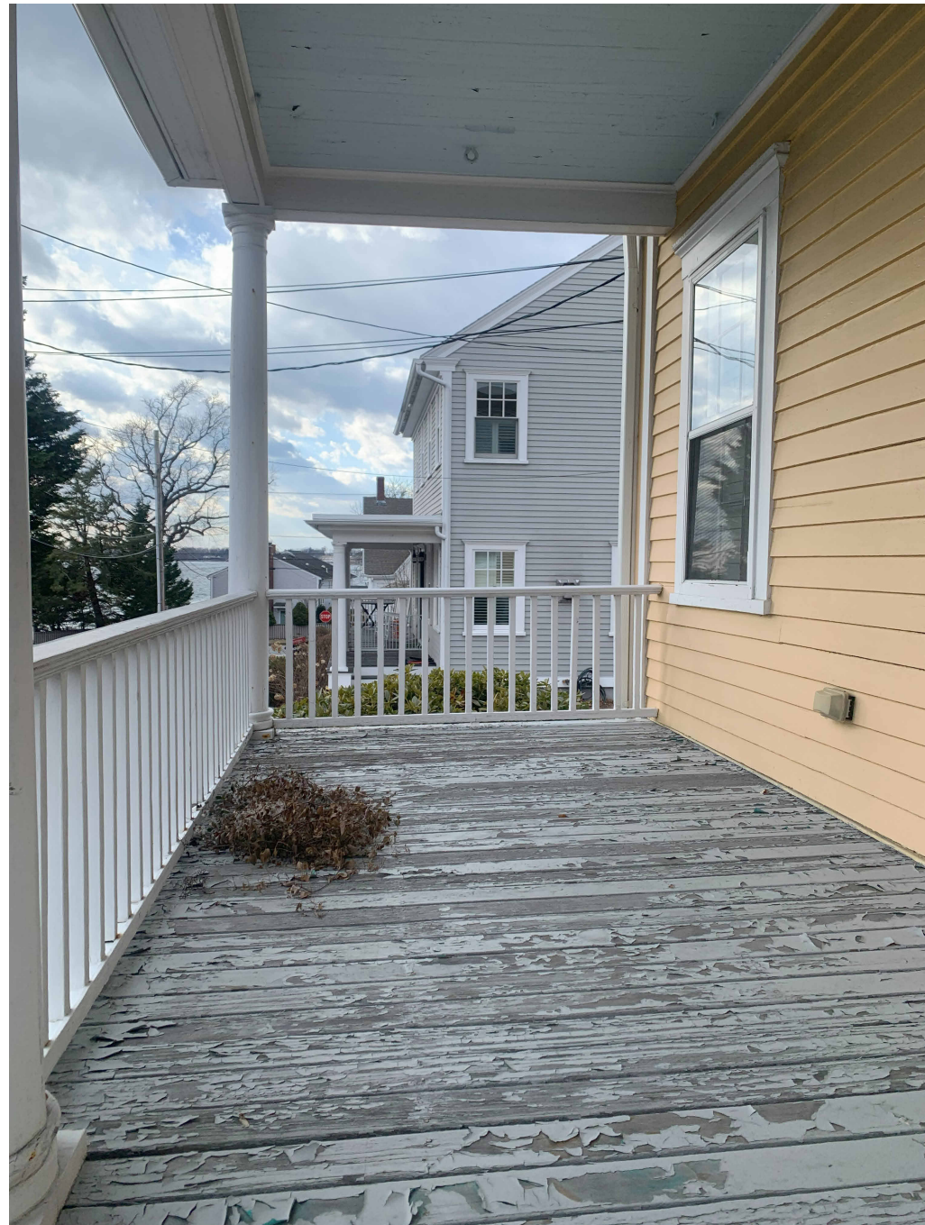
Photo #8: View of existing front porch decking
