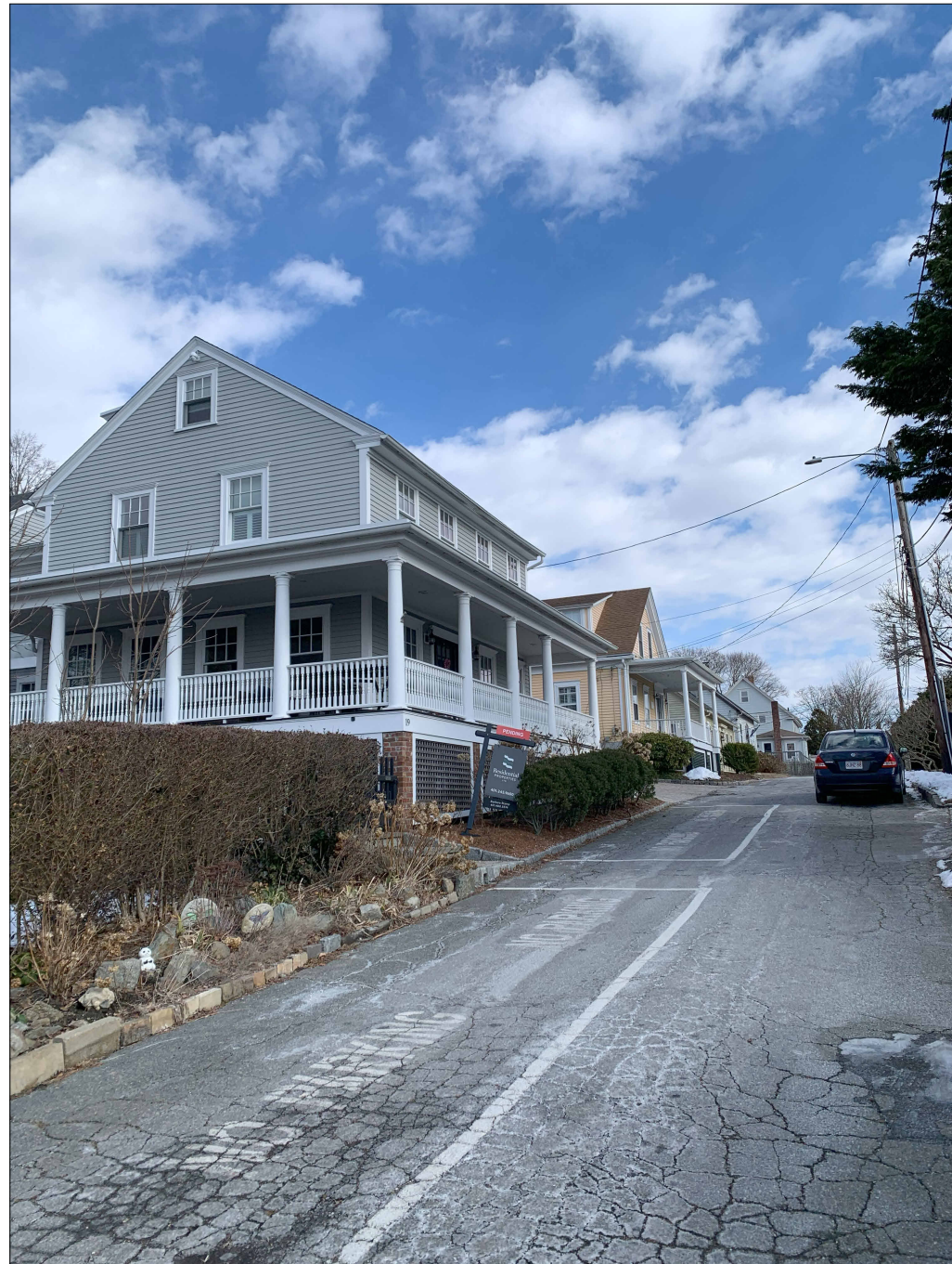
Photo #1: Front West side view, bottom of Summer Street
