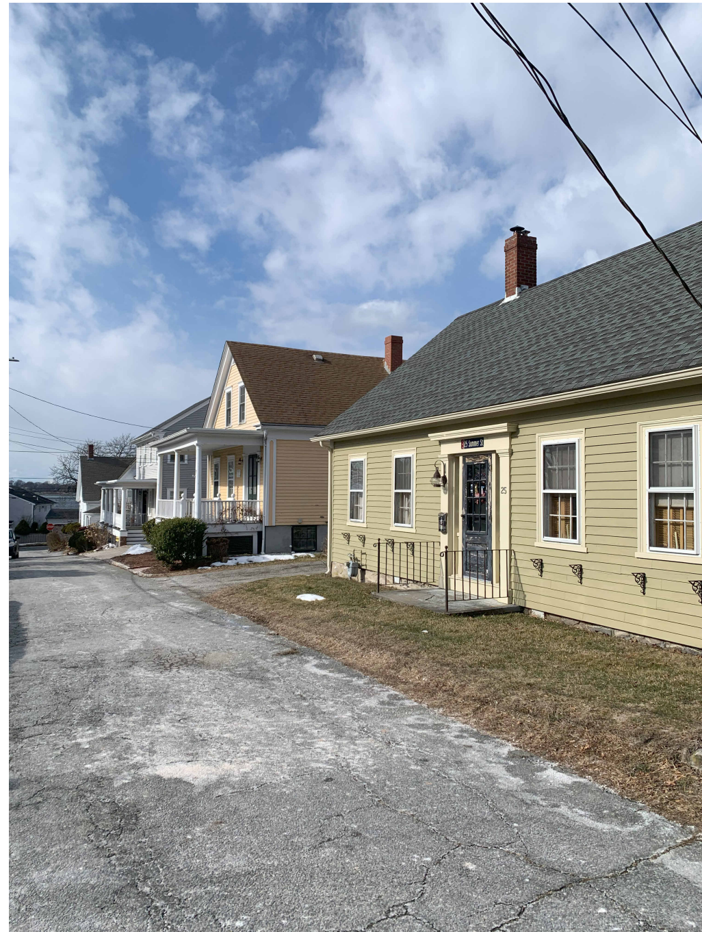
Photo #4: Front East side view, top of Summer Street
