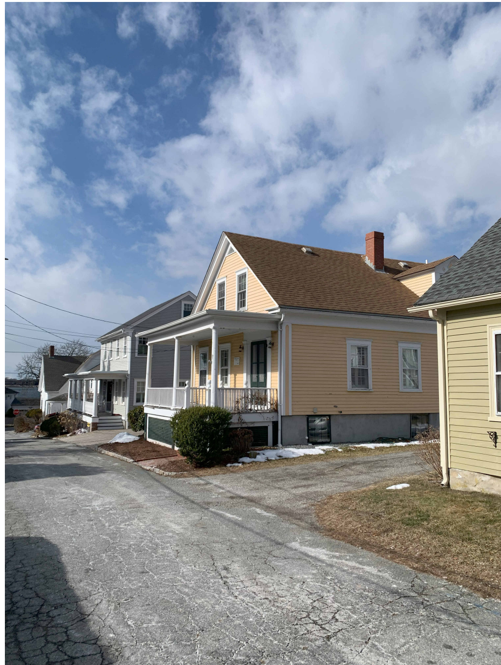
Photo #3: Front East side view, southeast corner of property
