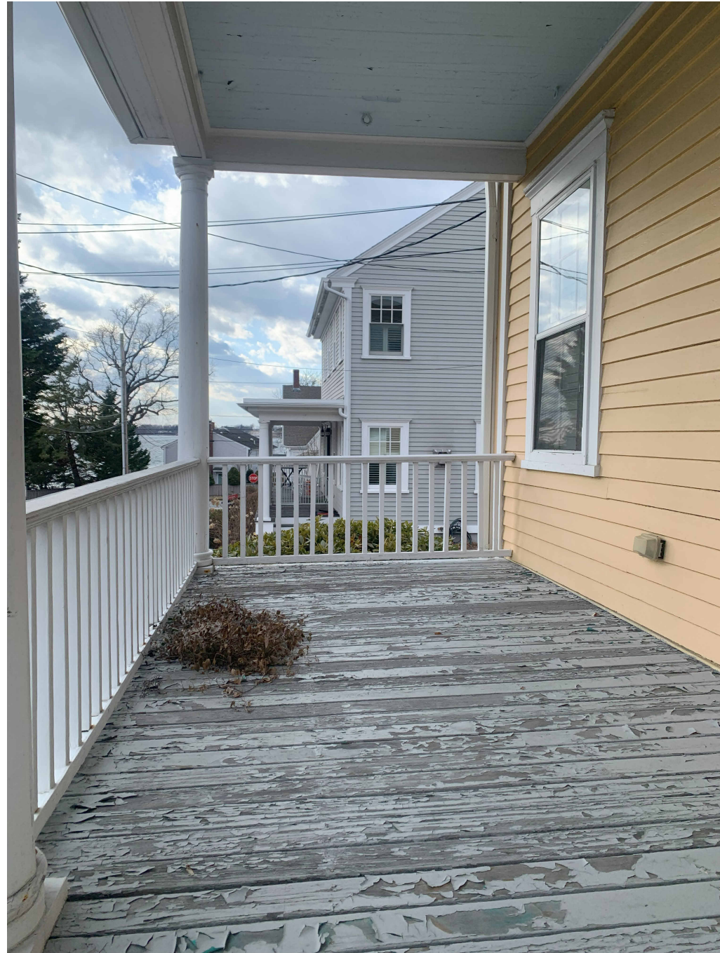
Photo #8: View of existing front porch decking
