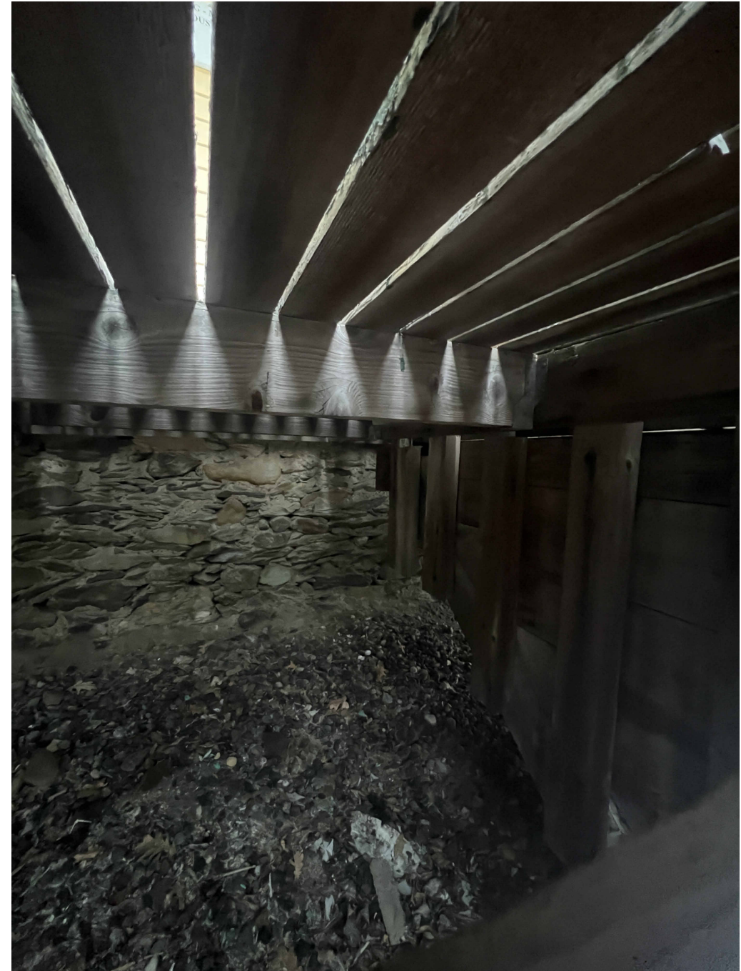
Photo #9: View of existing structure below front porch
