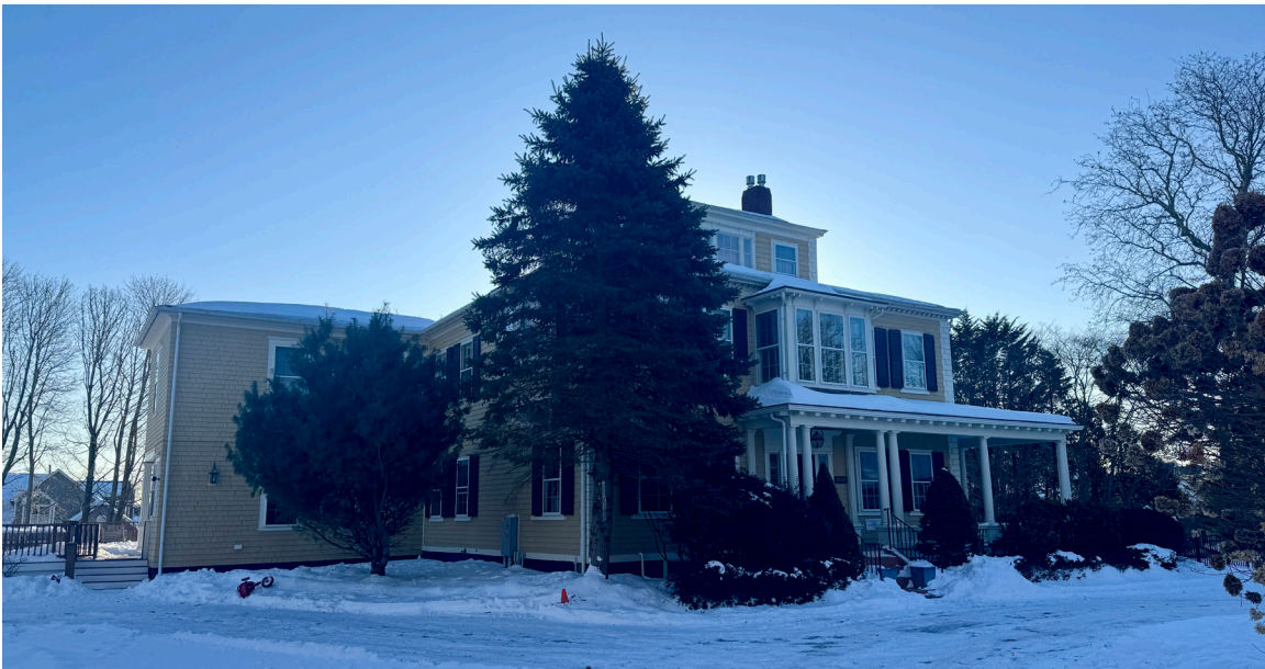
Existing house from driveway
