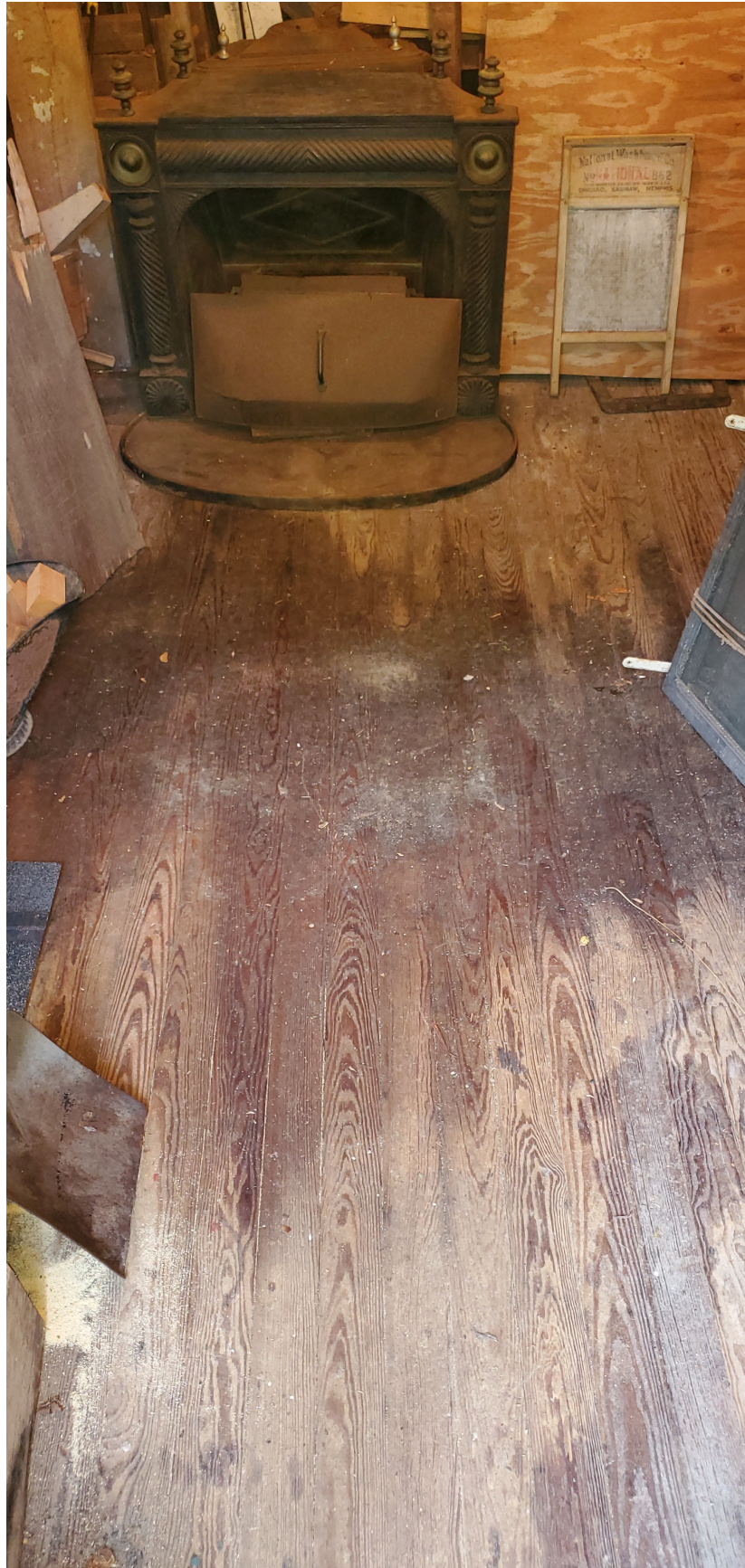
Figure 3: Carriage House first floor hard-wood floor boards
