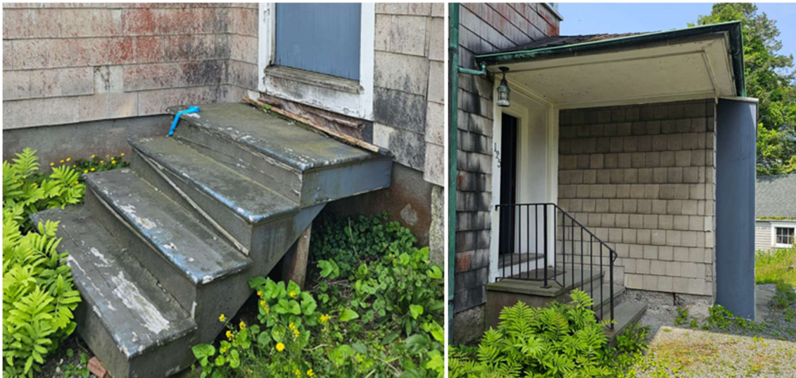
Images of both sets of exterior stairs facing the street.
