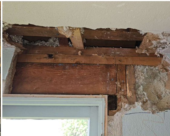
Image at second floor top plate & window header.
