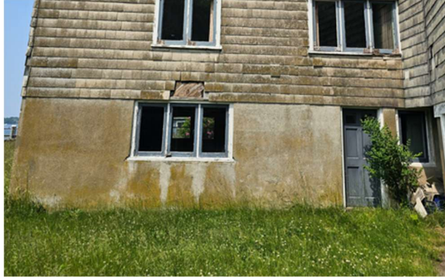
Image at rear of house, east facing foundation wall.
