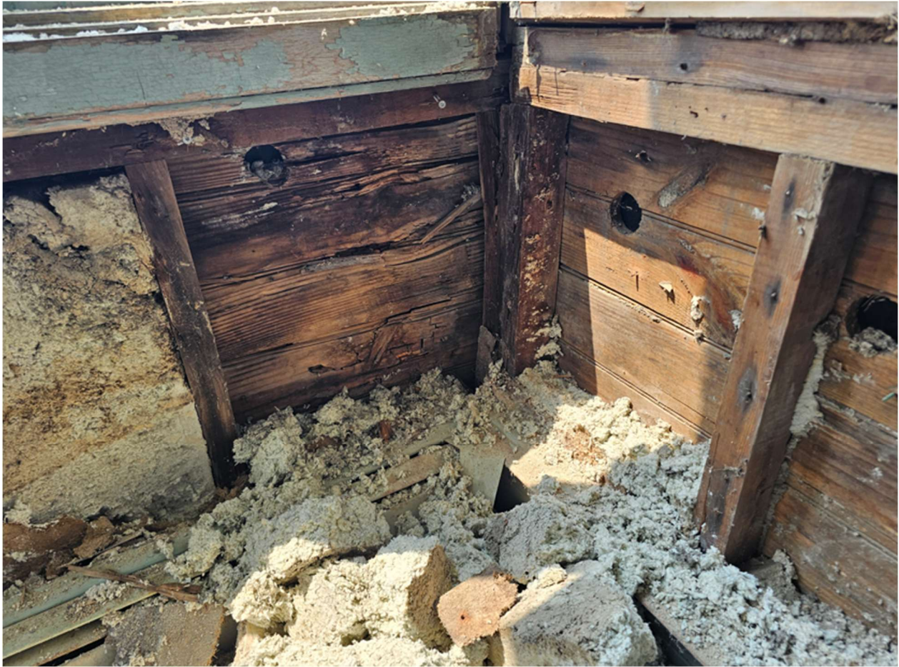
Image at second floor corner window sill framing.
