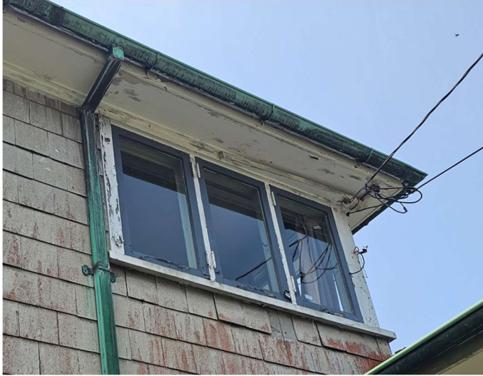
Image at second floor windows facing Hope Street.
