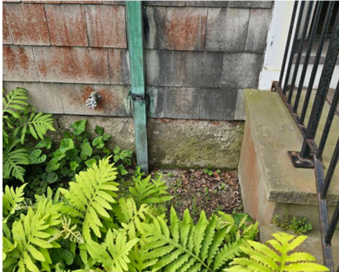
Image at street facing foundation wall.
