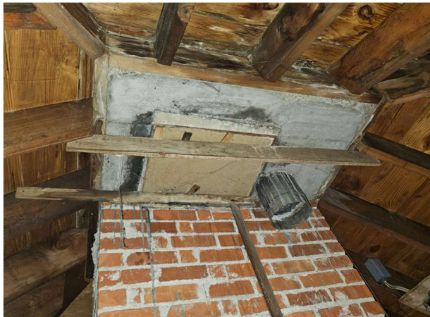
Image at main house chimney to roof connection.
