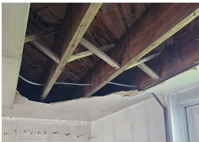
Image at first floor framing.
