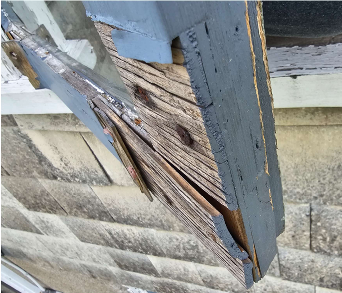
Image at side detail of second floor casement window patch.
