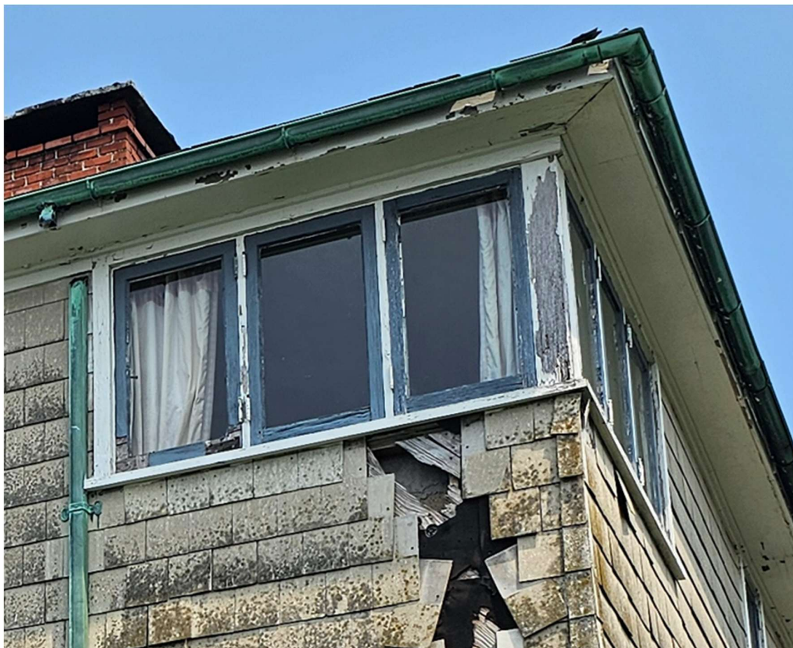
Image at second floor rear facing corner window.
