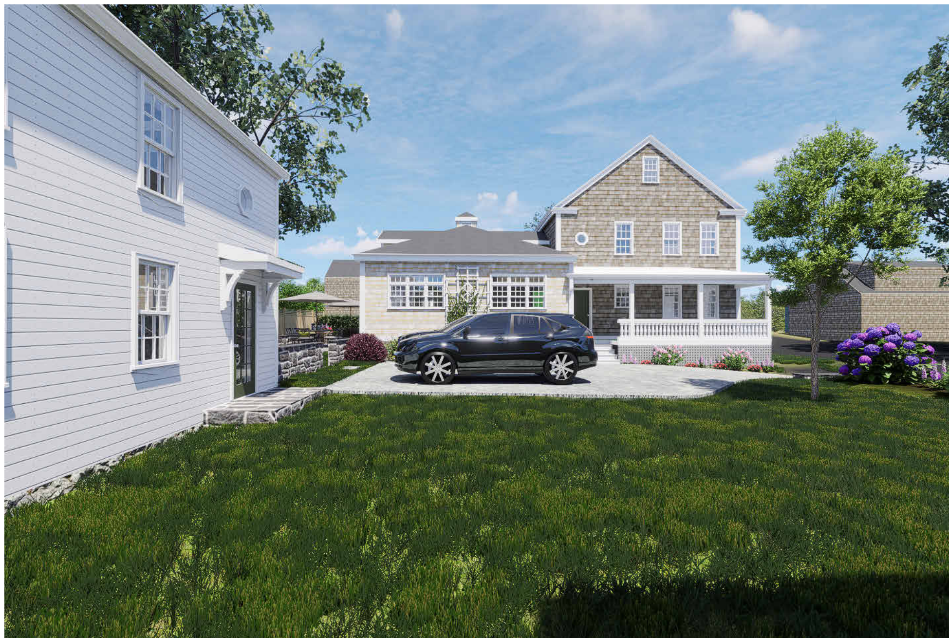
SIDE YARD VIEW
