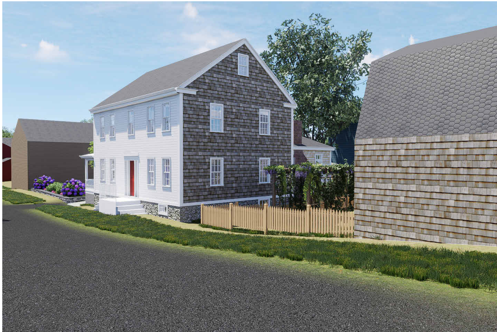
FRONT EAST SIDE VIEW
