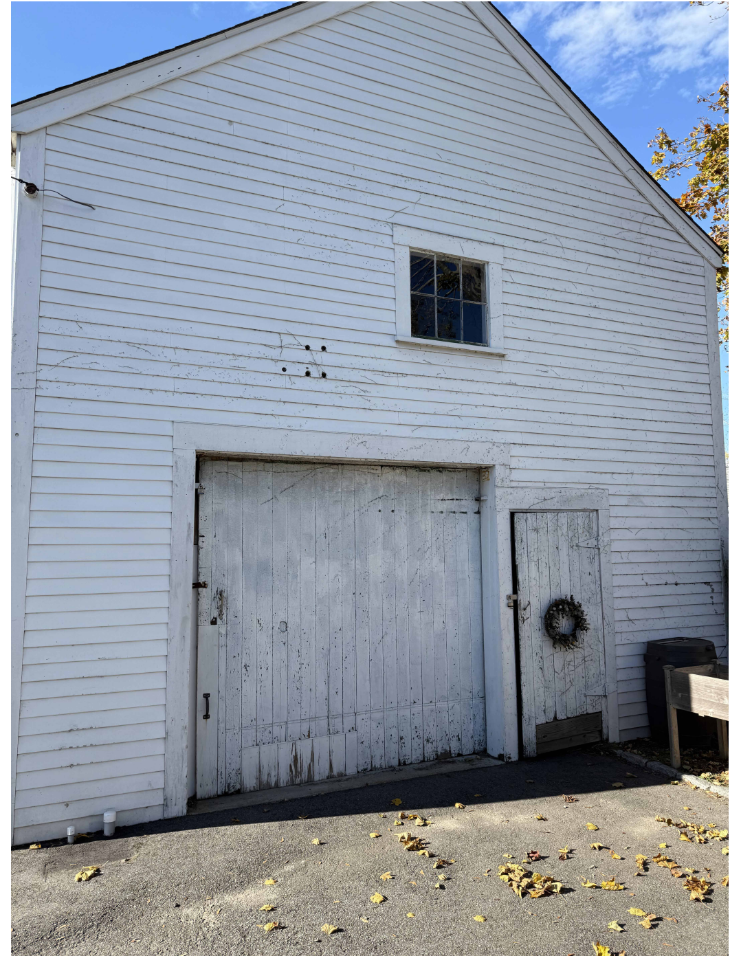
Photo #11: View of Eastern face of existing carriage house
