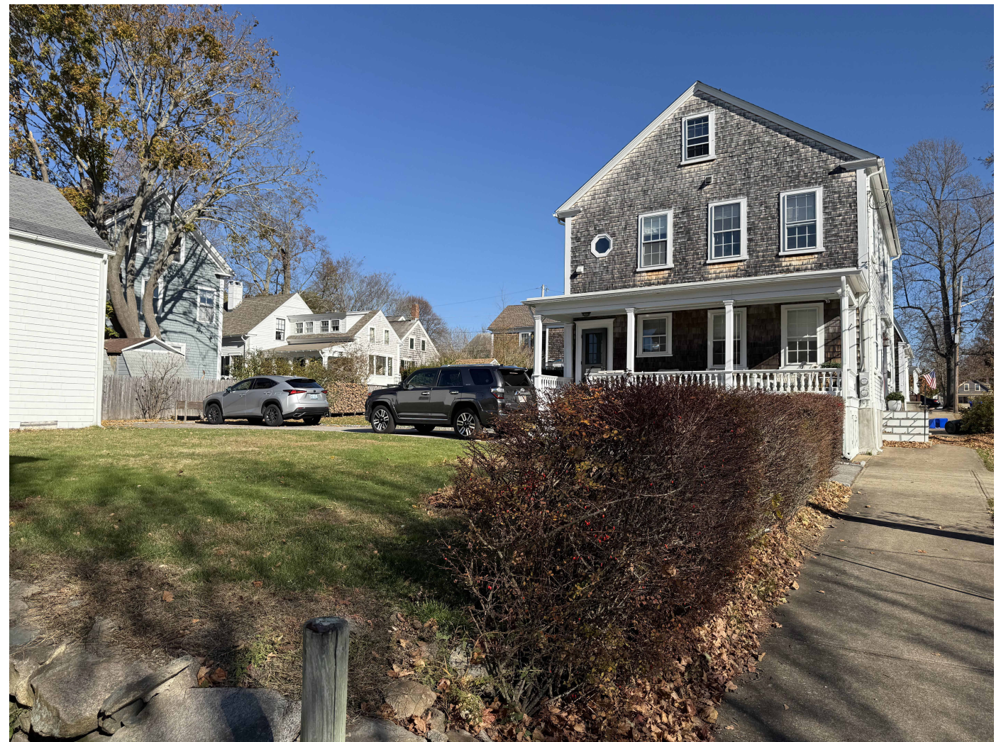
Photo #4: Front West side view, southwest corner of property
