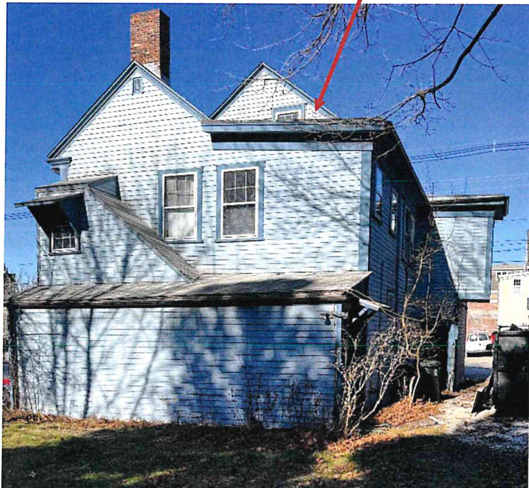
28 x 46 window 3 rd floor rear- Propose to change to casement- See spec on page 17
