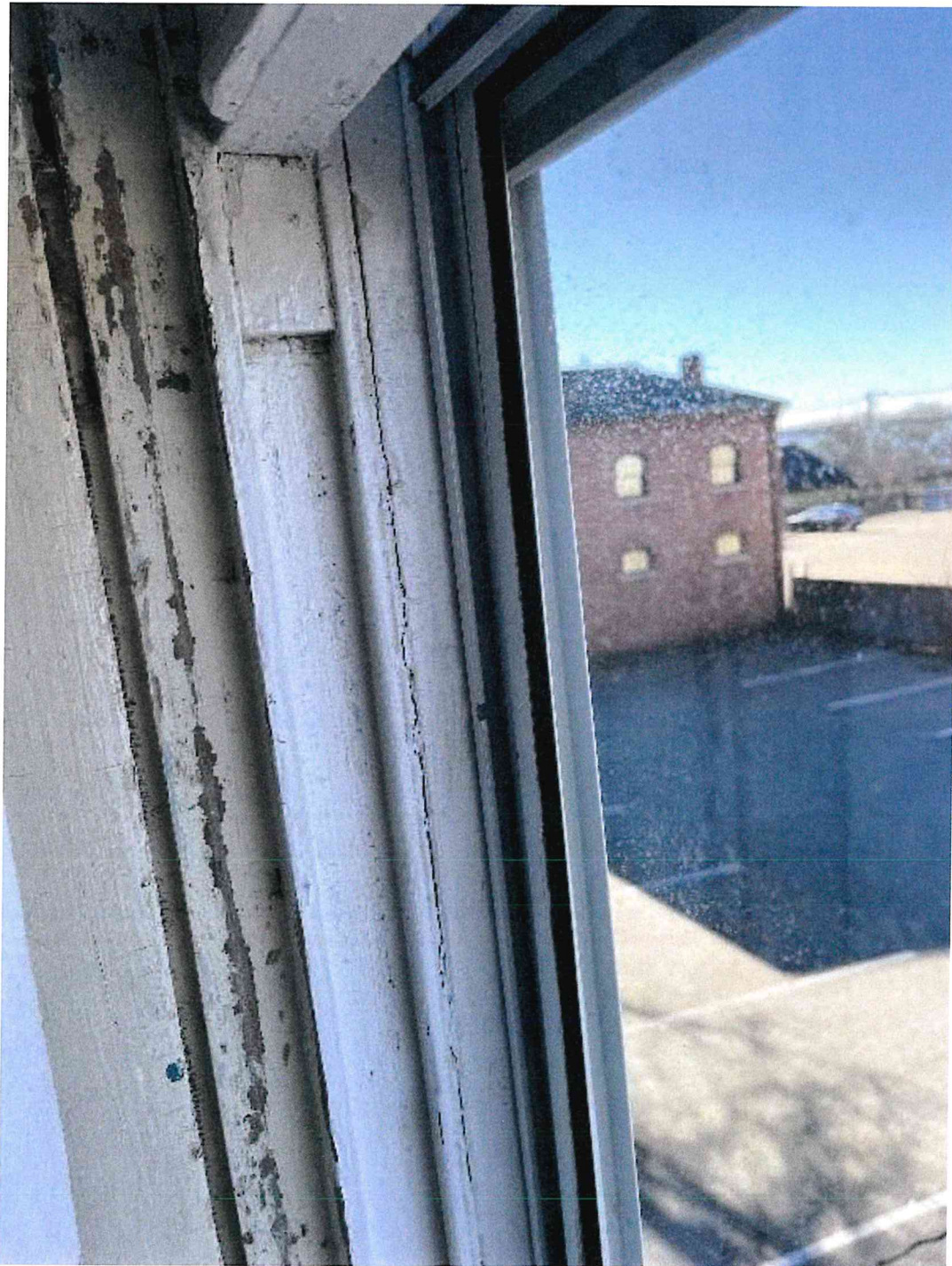
Location: 2 nd Floor West Side Top sashes on all window are fixed, preventing the window from opening
