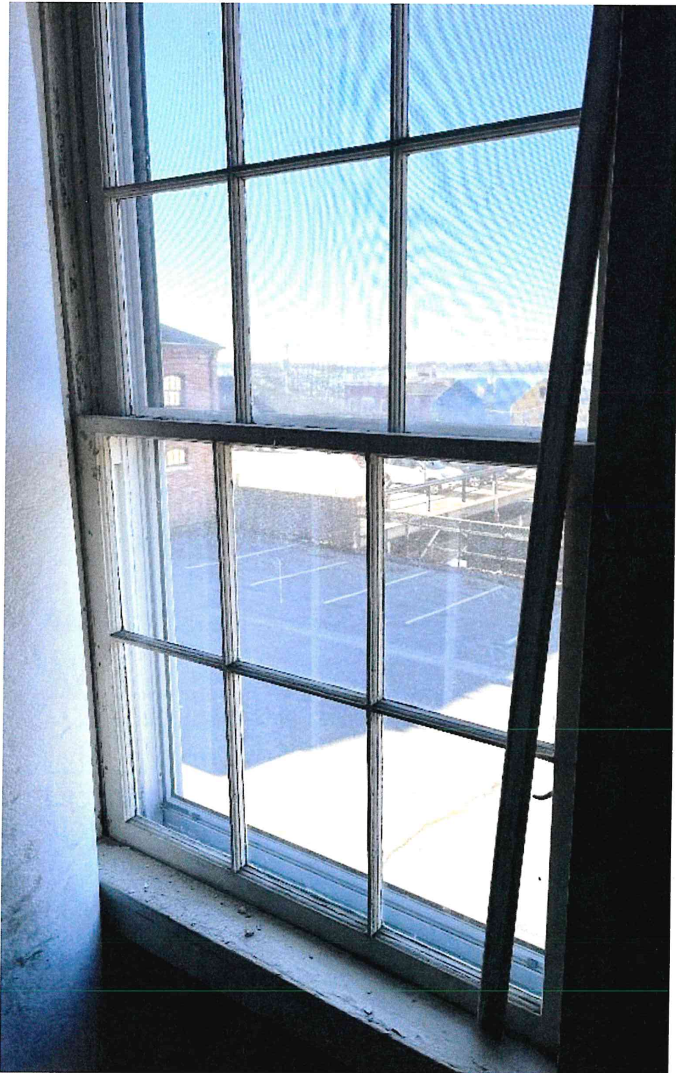
Location: 2 nd Floor West Side Many of the windows are missing window stops as seen above
