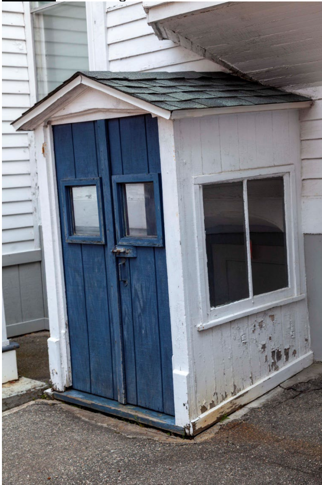
Photo 6 – Existing Bulkhead Enclosure
