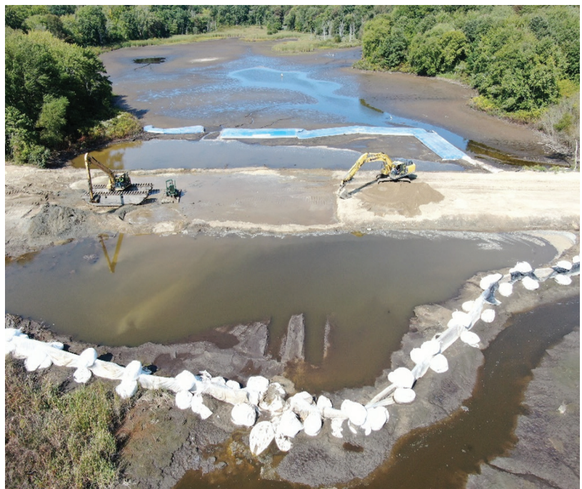
Construction work to remove the Upper Dam
