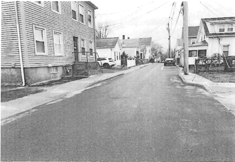
45 Congregational Street- westbound view 14' 6" curb to curb
