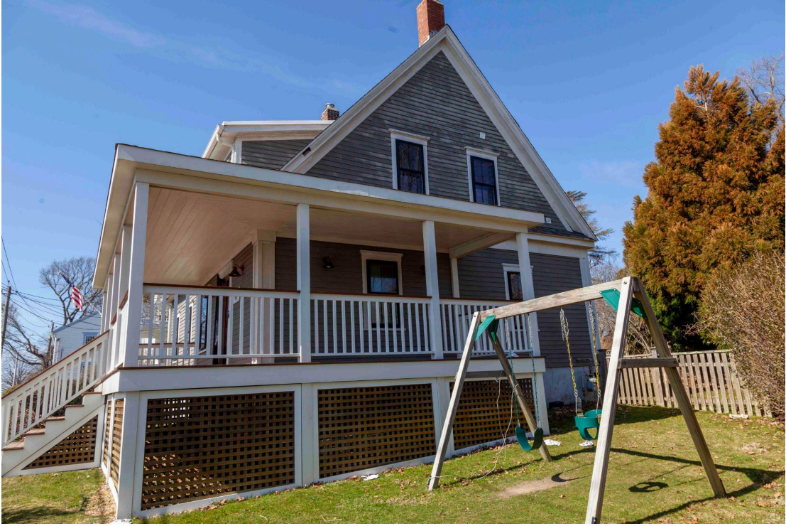
Photo 4 - Southeast View of the Existing Residence
