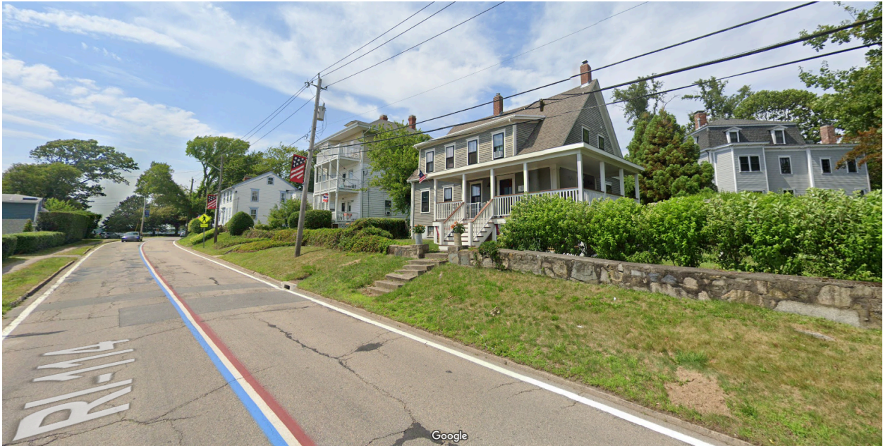
Photo 9 - The House with Street Context Shown (Google Street View July 2023)
