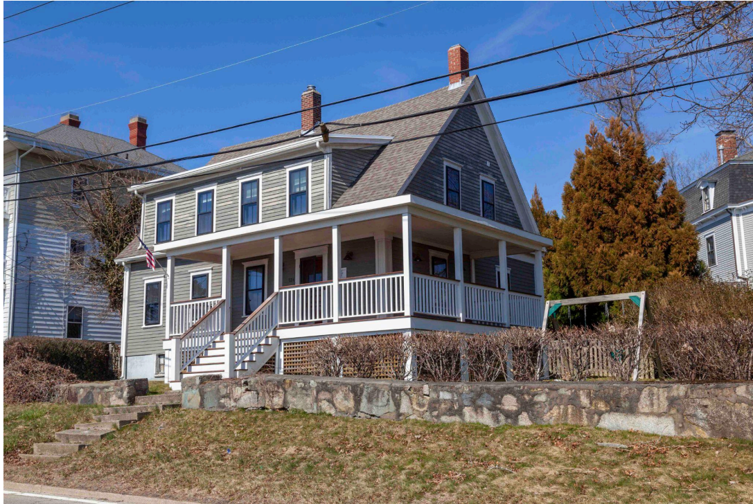
Photo 1 - South View of the Existing Residence
