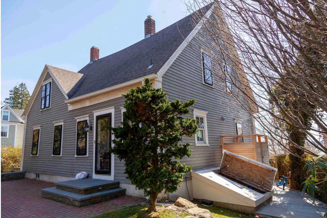
Photo 6 - Existing Portions Roof to be Removed for Dormer
