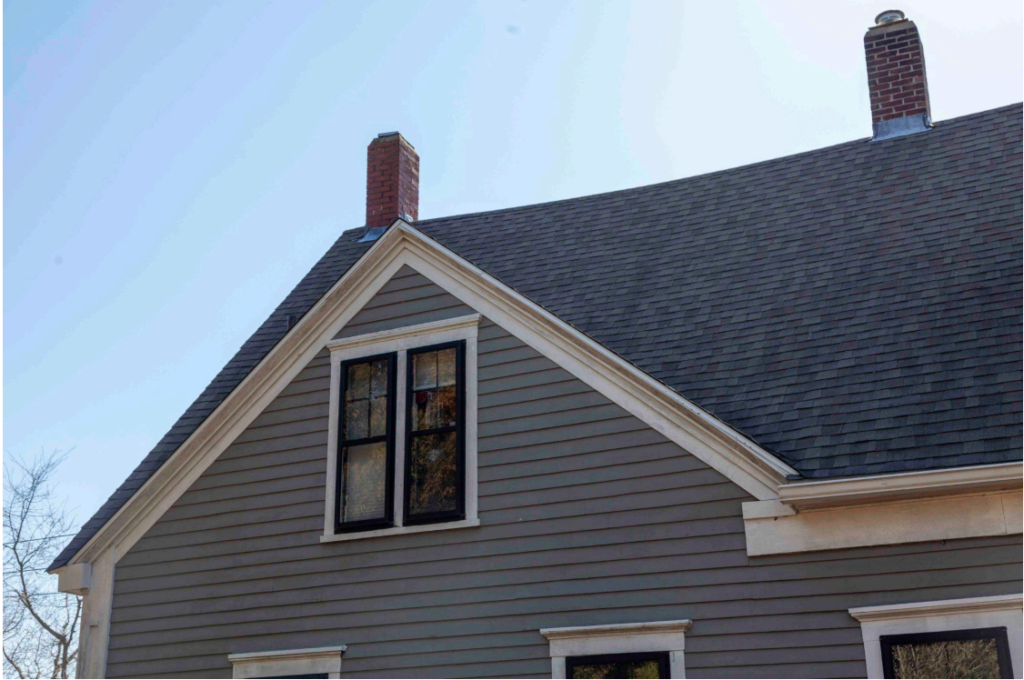
Photo 5 - Existing Gable to be Removed. Window to be Removed and Stored
