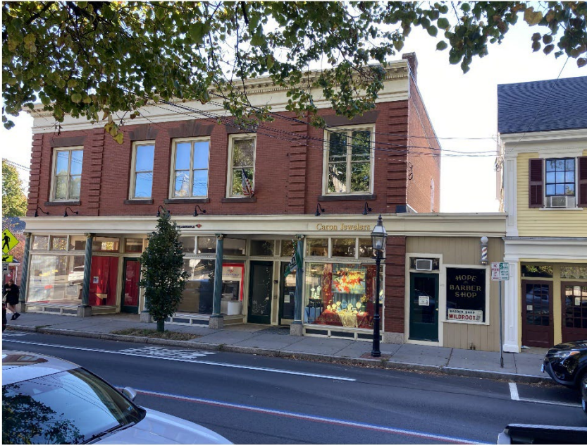
Photo 1 – Existing Hope Street Facade
