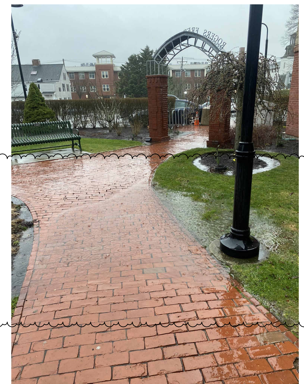
IMAGE OF WATER COLLECTING AT THE BRICK BRICK PATH AT SEATING AREA.
