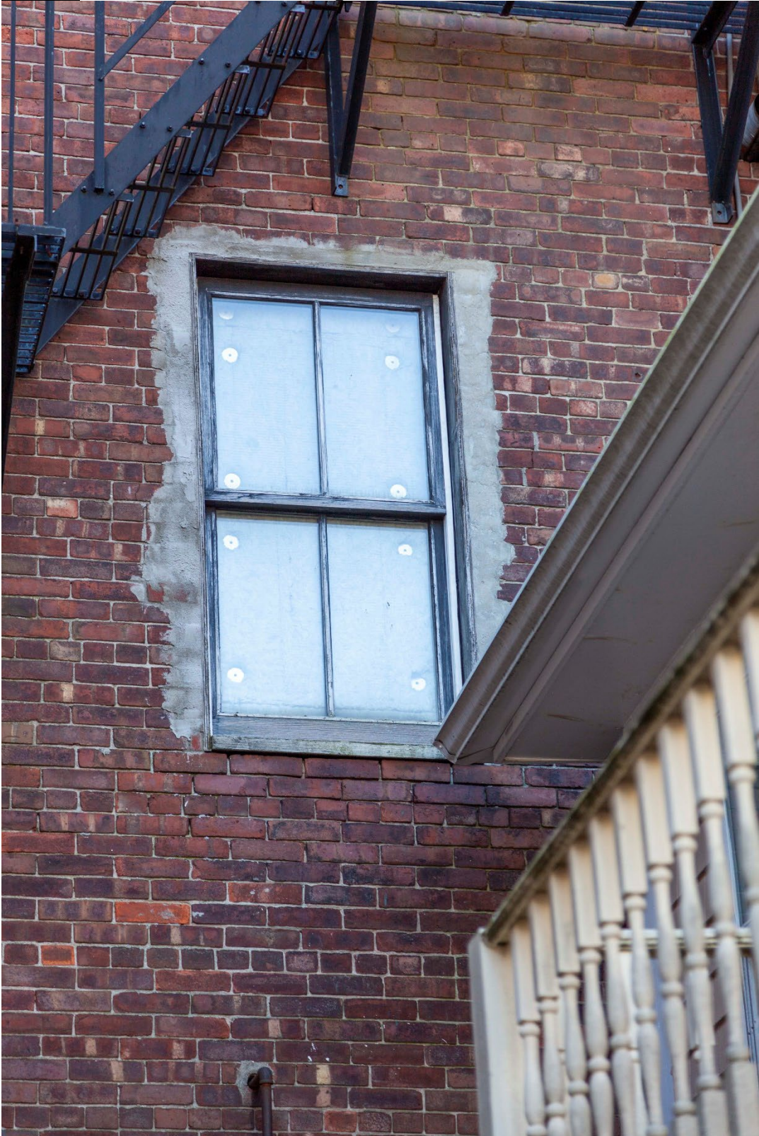
Photo 8 – North elevation showing window to be restored.
