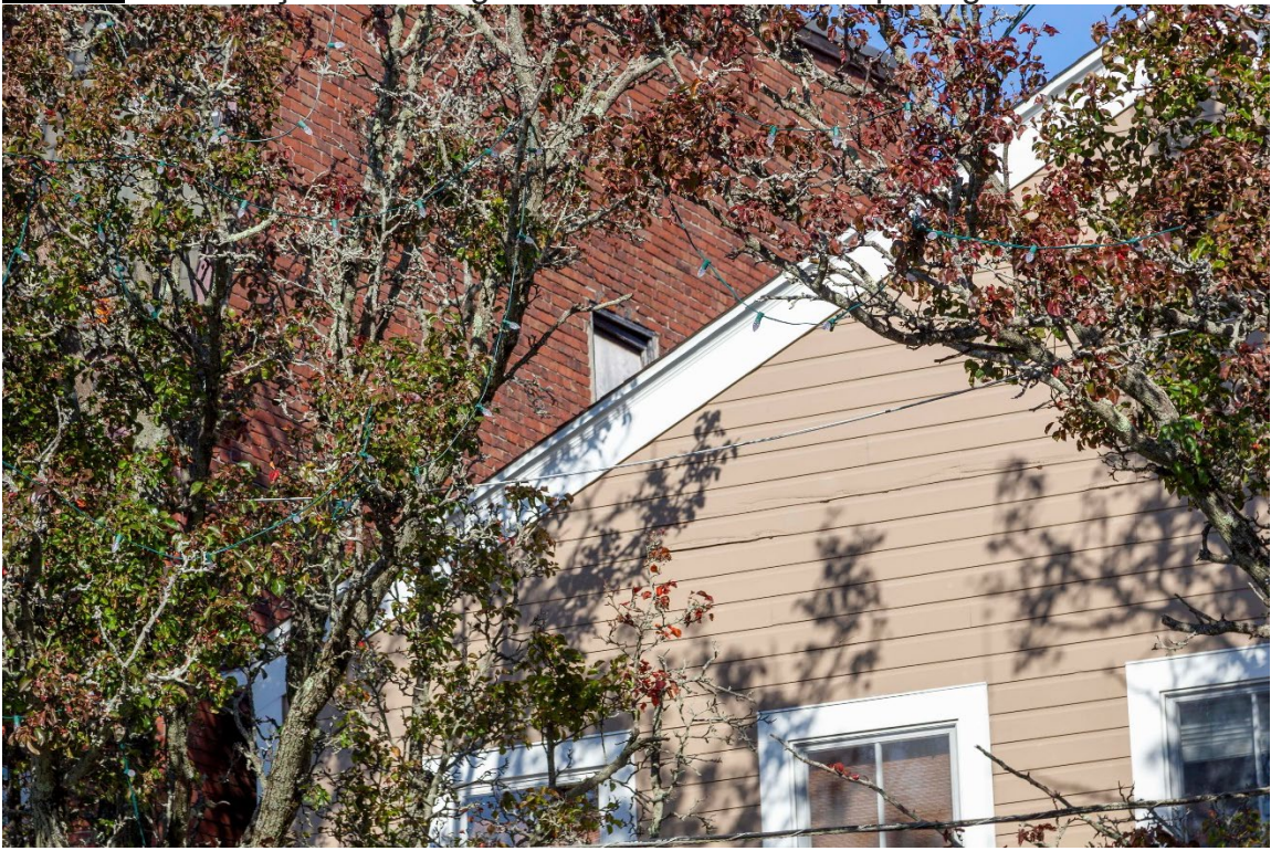
Photo 7 – East façade showing visible view of window opening to be restored.
