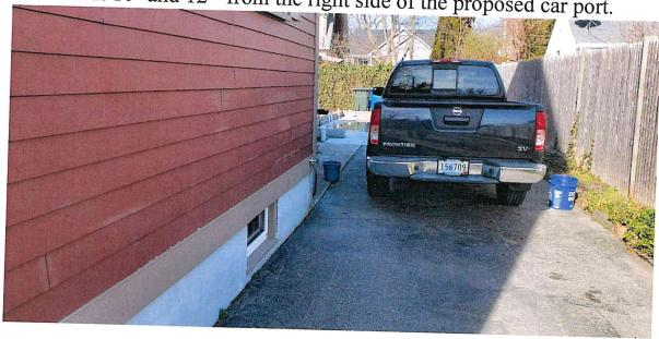
Original Proposed posts Buckets are 10' apart per original plans, you can see the bucket on the left is in the line of travel when you back out of the garage.
