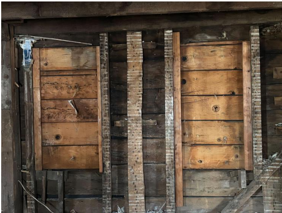
Evidence of original windows along the right side of the house that were previously boarded up. 6 on 1st floor, 6 on second floor. Proposing to reinstall with matching Pella wood clad 6/6 double hung windows. Same size and style windows as the left and rear sides.
