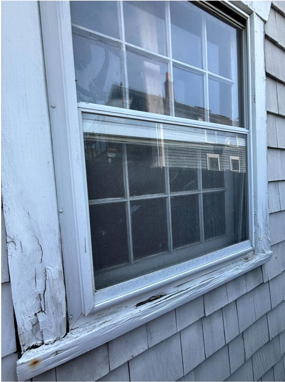
View of one of many rotted windows in poor condition.
