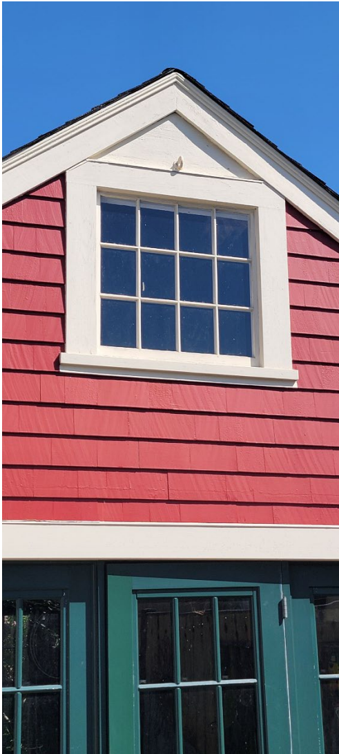
Photo #5: Second Floor fixed 12-lite fixed window
