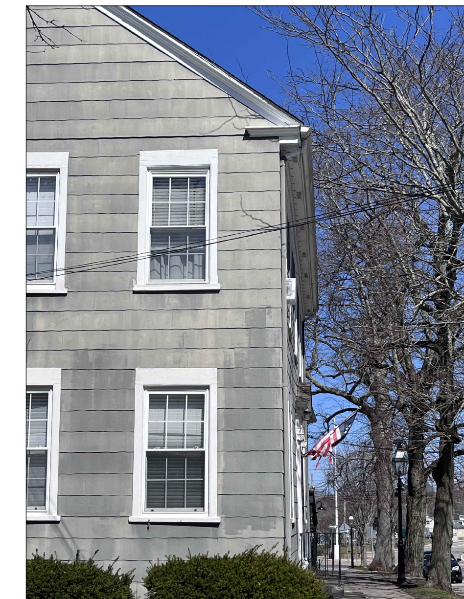
05 CORNICE RETURN ON EXISTING HOUSE SCALE: N/A
