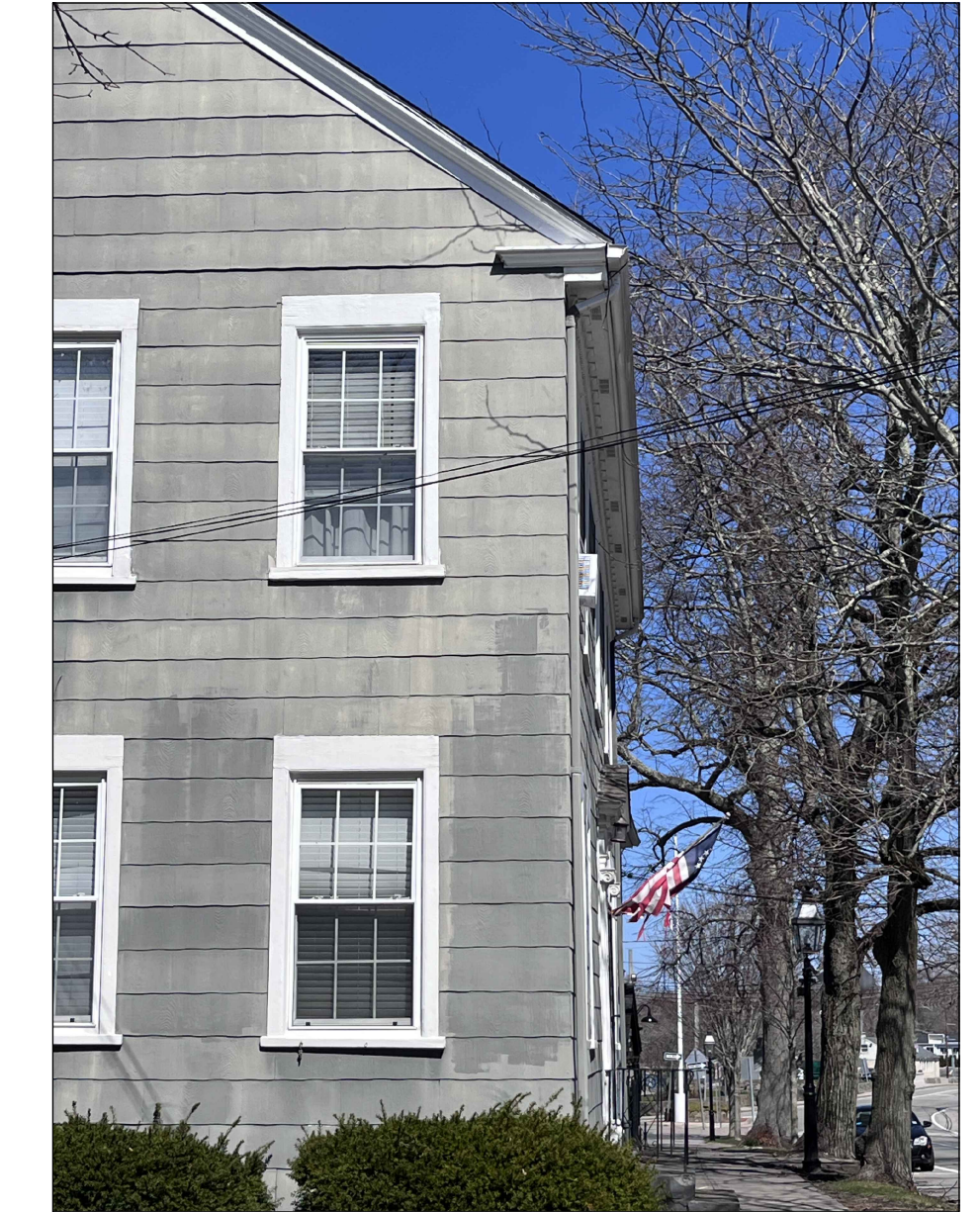
05 CORNICE RETURN ON EXISTING HOUSE SCALE: N/A
