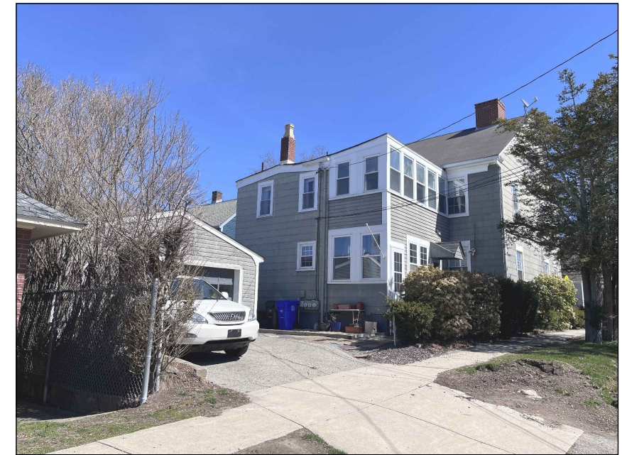
04 PRIMARY STRUCTURE FROM OLIVER ST SCALE: N/A
