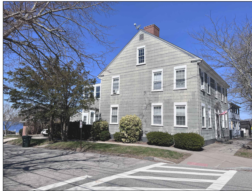
03 PRIMARY STRUCTURE FROM OLIVER ST SCALE: N/A
