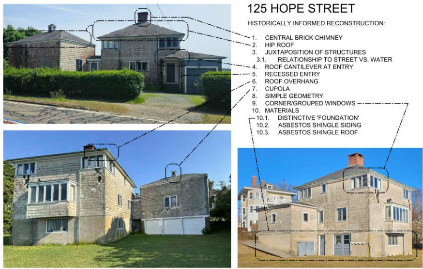
Figure 1. Existing house with character-defining features identified.
