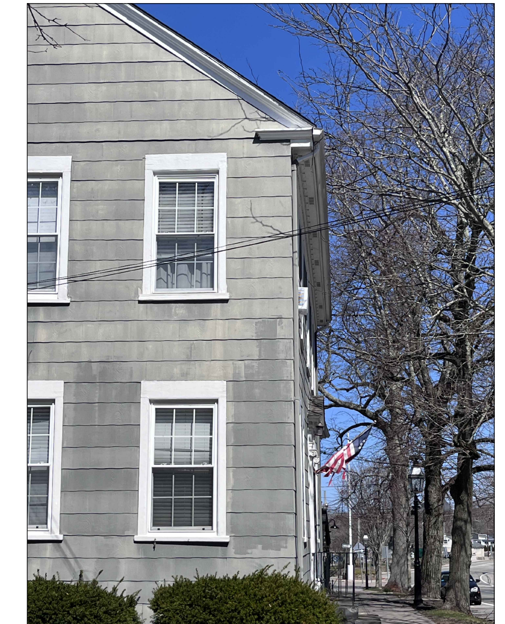
05 CORNICE RETURN ON EXISTING HOUSE SCALE: N/A
