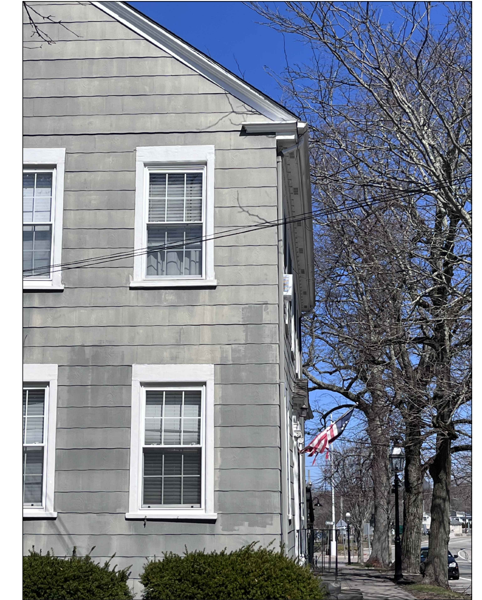
05 CORNICE RETURN ON EXISTING HOUSE SCALE: N/A
