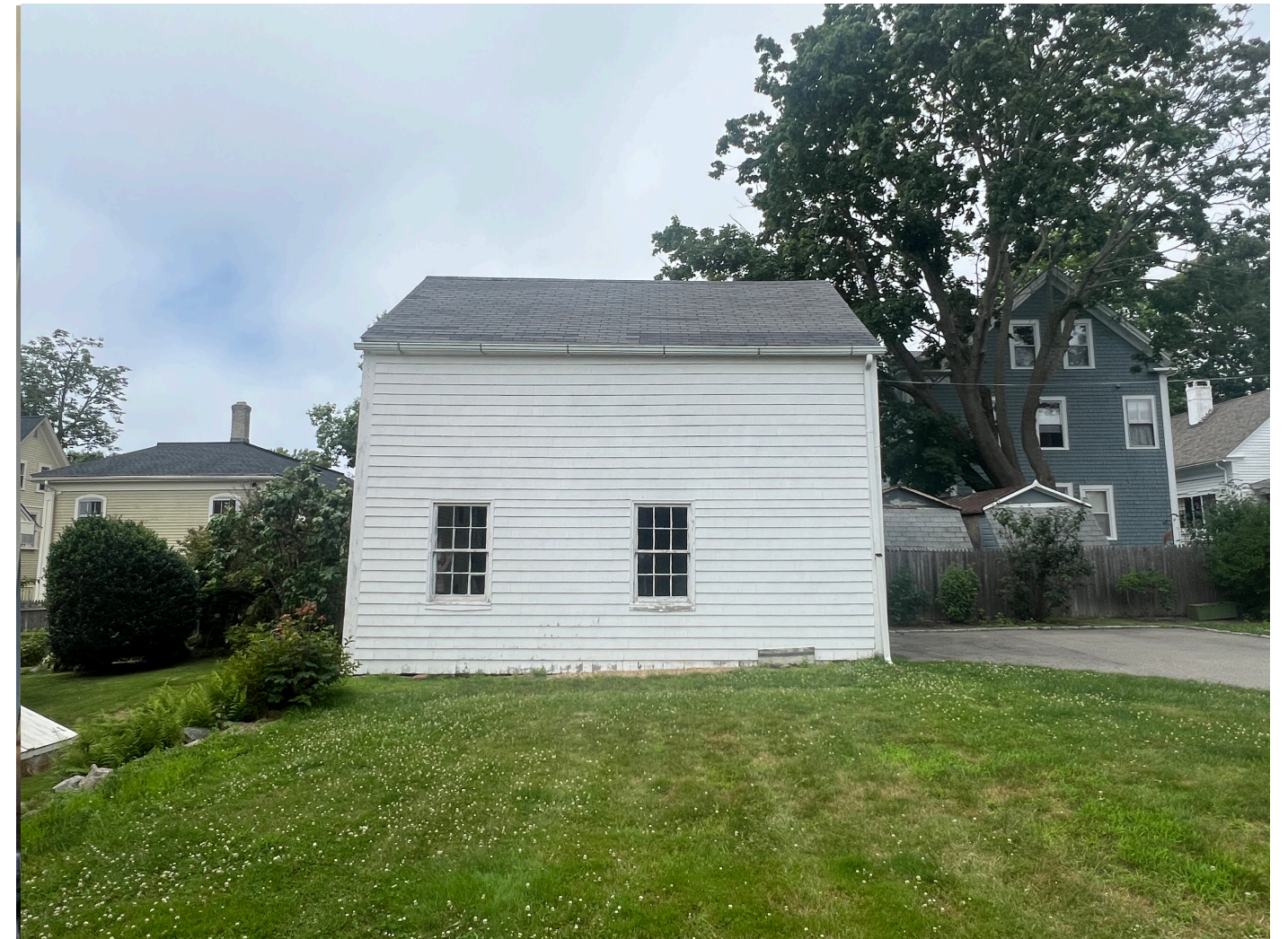
View 2: From front yard, looking north at carriage house south facade
