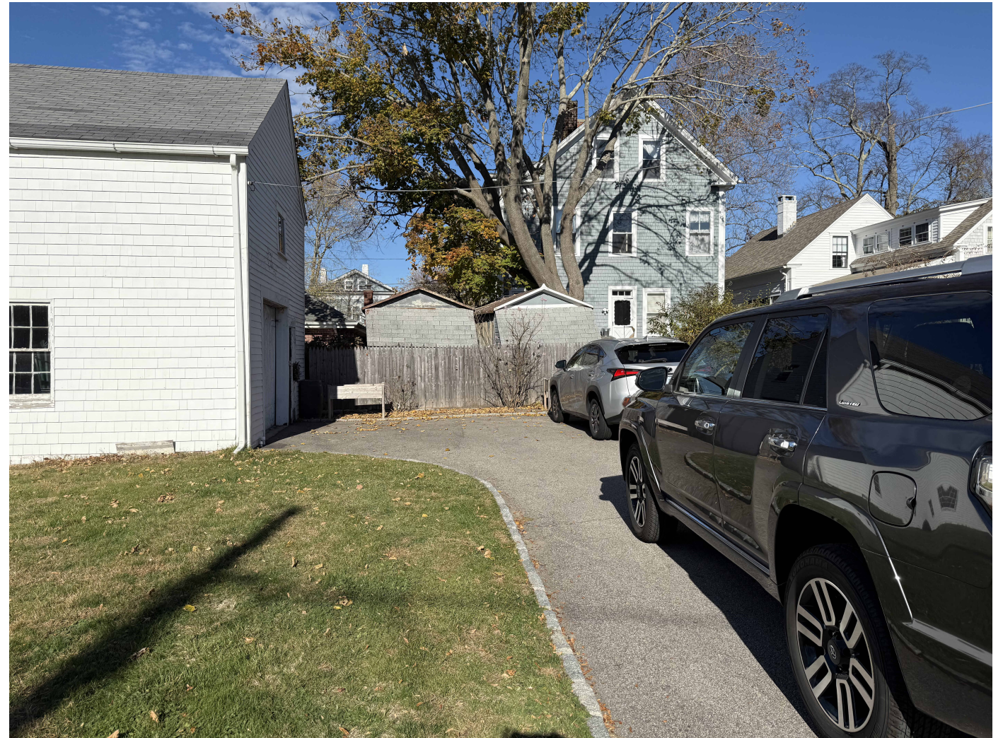
View 4: From front yard, looking north at carriage house and driveway
