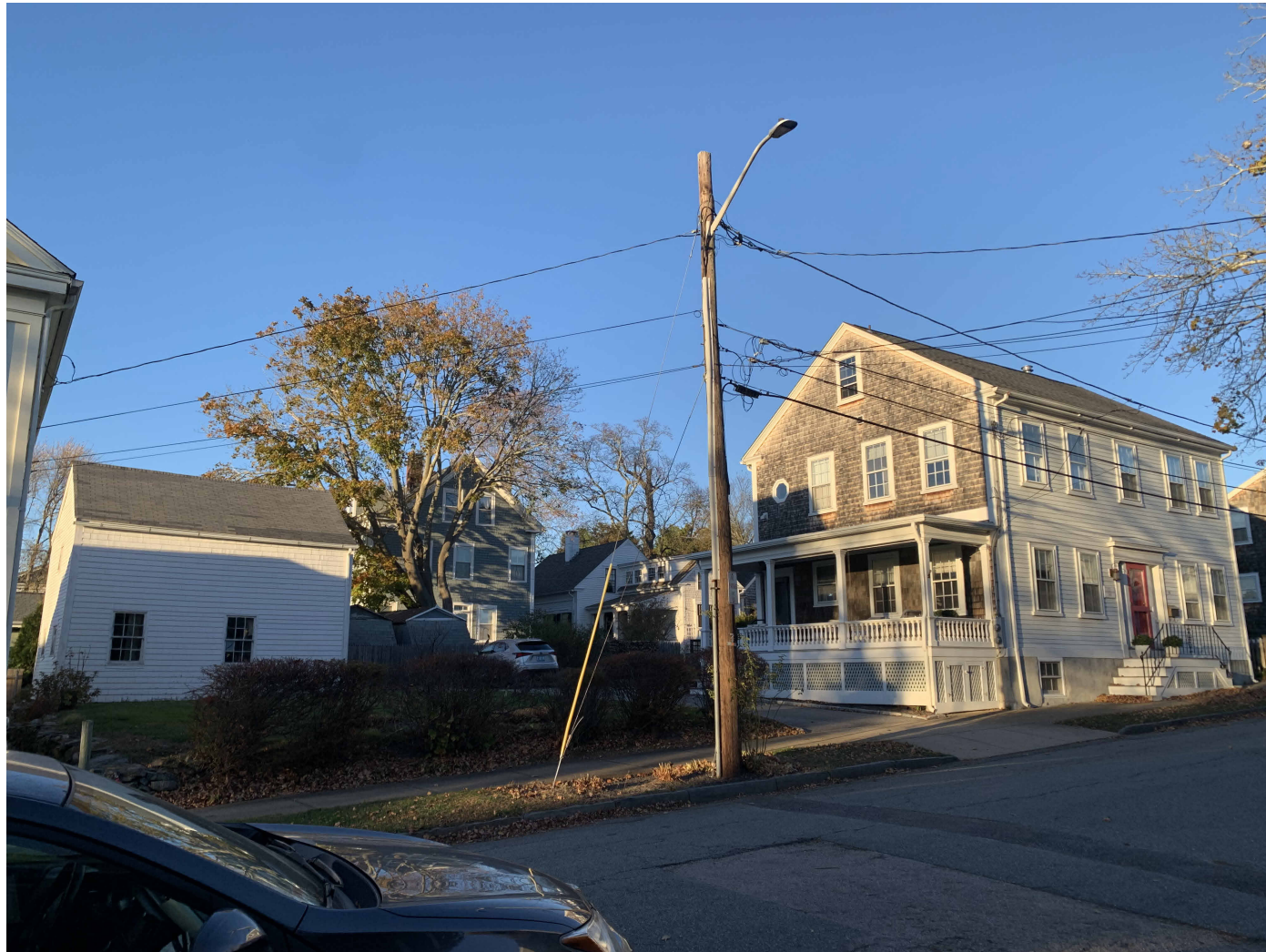
View 1: From Byfield Street, looking northeast at 19 Byfield property
