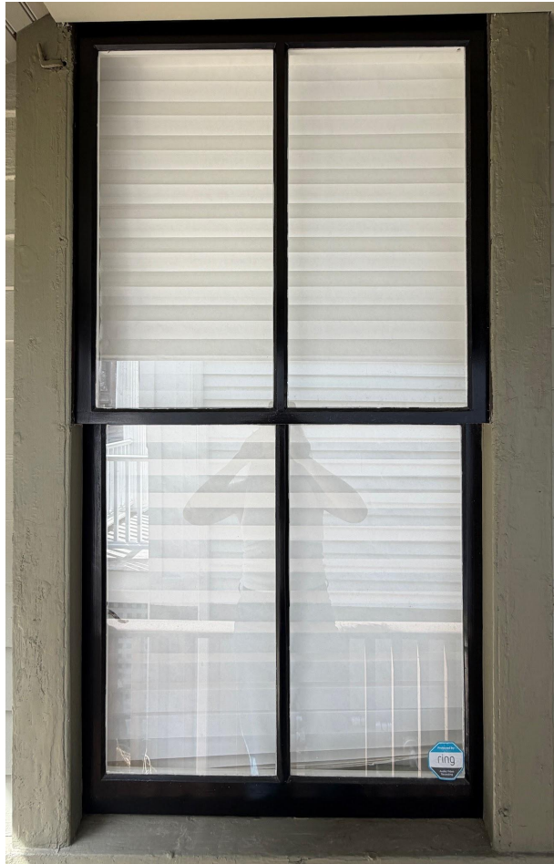
Window 1A (right side, 1st floor)
