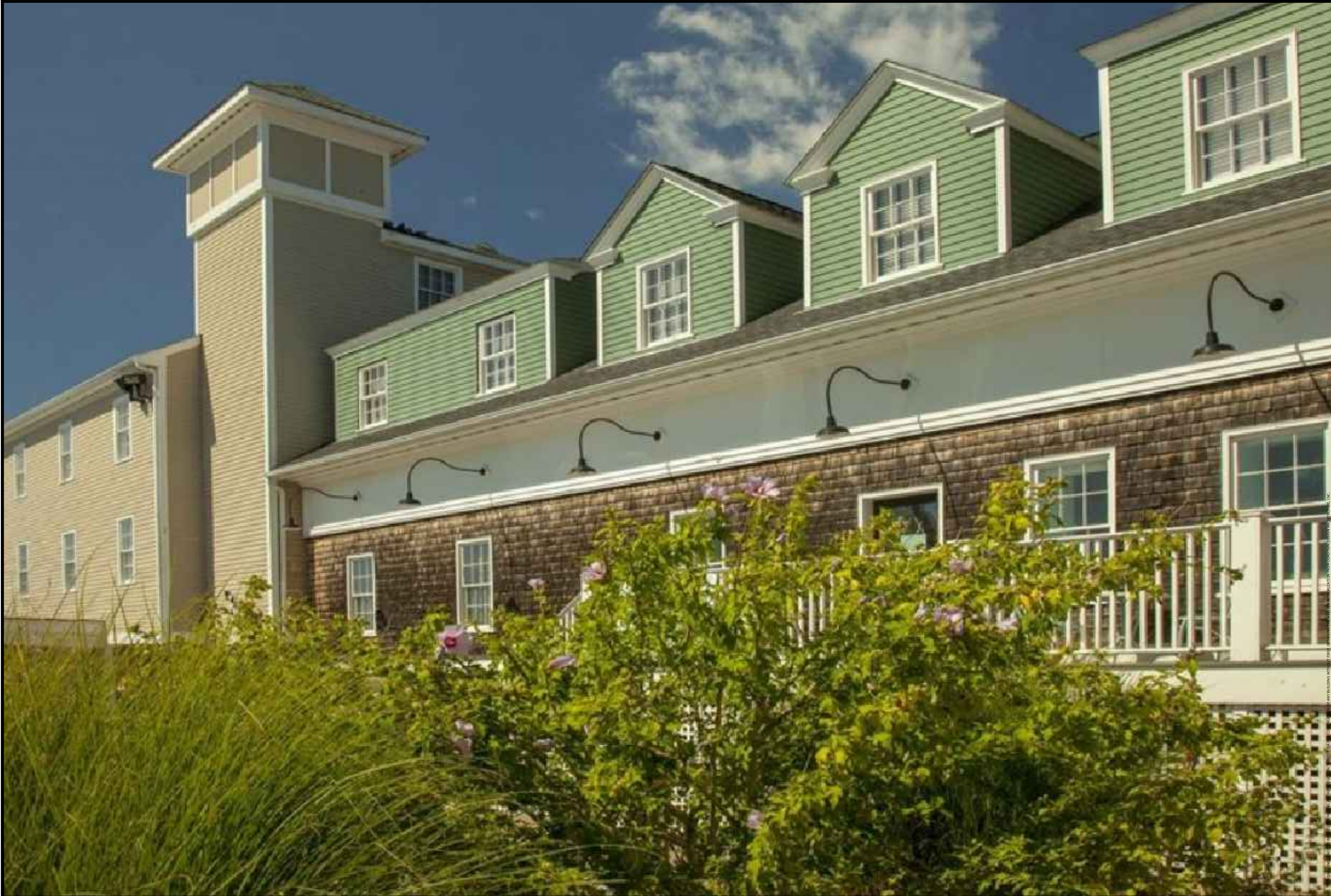
① EXTERIOR PHOTO 2
