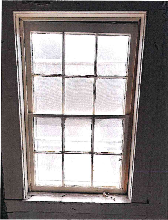
28 x 46 window 3 rd floor rear- Propose to change to casement- See spec on page 17
