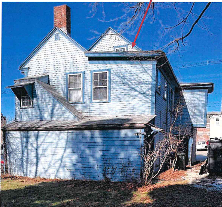
28 x 46 window 3 rd floor rear- Propose to change to casement- See spec on page 17
