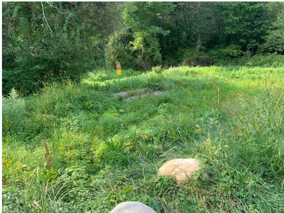
Photo No. 1: Vegetative growth within Spillway
