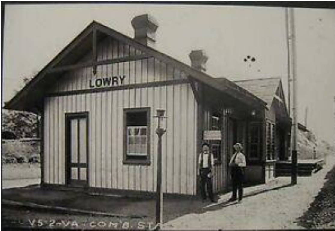
Lowry, VA Train Depot - 1890
