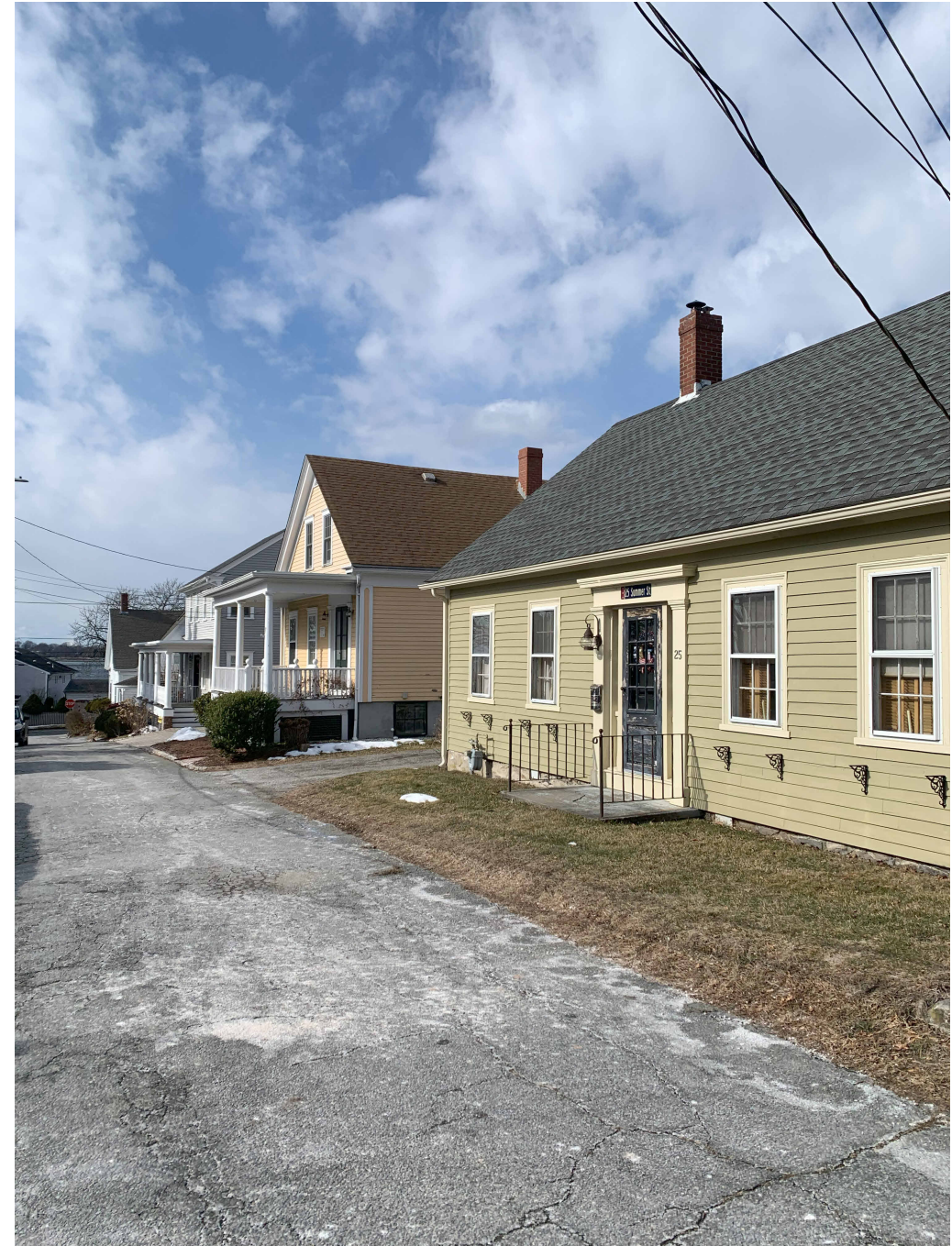
Photo #4: Front East side view, top of Summer Street
