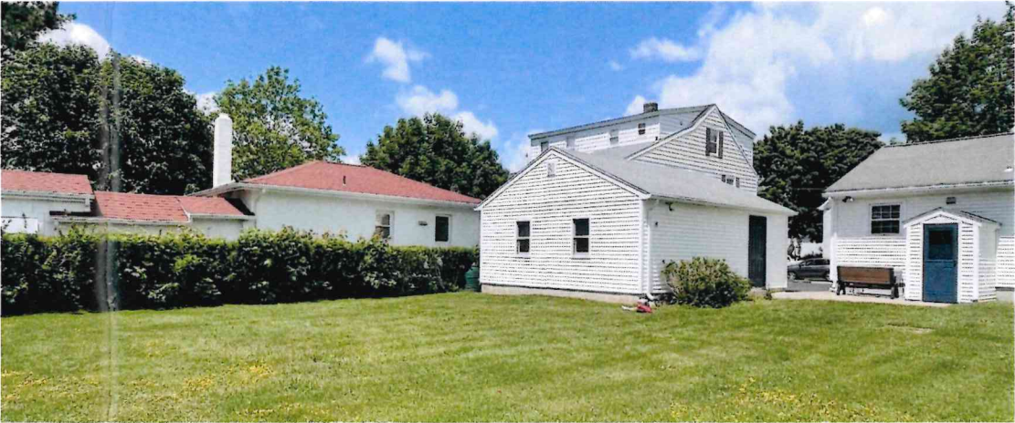
EXISTING PHOTOS OF HOUSE NEXT DOOR AND LOCATION OF PROPOSED ADDITION
