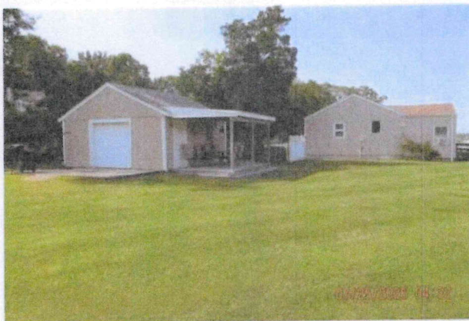
Cottage & Garage - to be demolished
