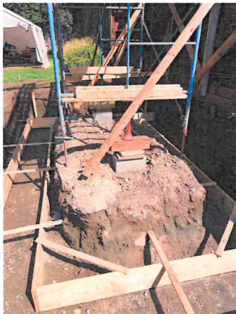
Excavation for footing
