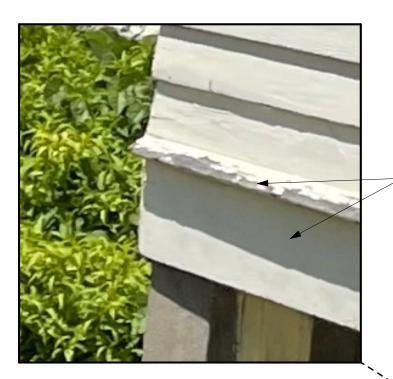
WATER TABLE -CEDAR WOOD 10" BOARD WITH 1" WOOD OVERHANG (TOP) AT 45-DEGREES. TYP. EAST ELEVATION.
