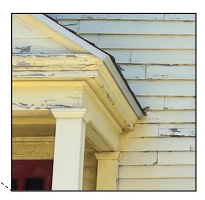
DETAIL AROUND FRONT ENTRY - REPAIR EXISTING WITH CEDAR WOOD, MATCH EXISTING SIZES & CONFIGURATIONS, REPAINT.
