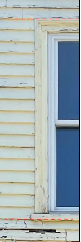
1X4 WOOD CEDAR TRIM @ JAMBS & HEAD, 1 5/8" SILL AT BOTTOM, EXTENDING 1" BEYOND 1X4 @ JAMBS.. MODIFY/ADJUST SIDING EXPOSURE TO BEST FIT AROUND WINDOW, MATCHING **BOTTOM OF** COURSE TO BOTTOM OF SILL AND BOTTOM OF COURSE TO TOP OF WINDOW TRIM, TYP (SEE RED LINES).
