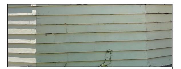
CEDAR CLAPBOARD SIDING +/- 4" EXPOSURE WITH MITERED JOINTS AT ANGLED WALLS.
