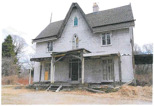
**Photograph No. 3:** Photograph taken on March 24, 2018, Photographer facing East The porches and much of the exterior is in very poor condition and planned for restoration/reconstruction.
