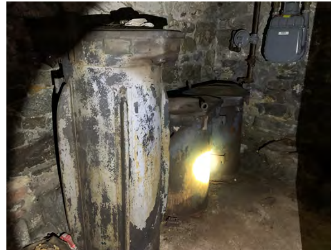
18. Suspect PCB-containing transformers stored in the basement in Building 1.
