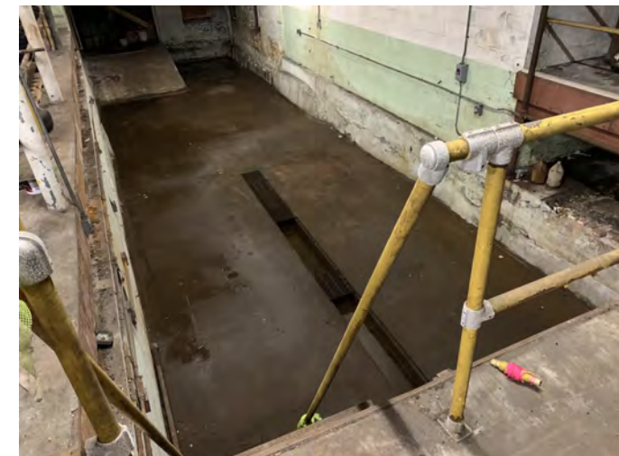
22. Floor drain trench associated with dye kettle observed in Building 5.
