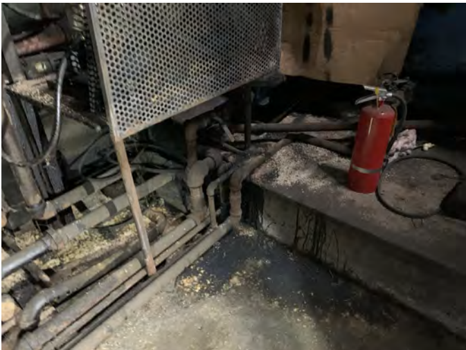
36. No. 6 oil staining observed on floor in Boiler Room.
