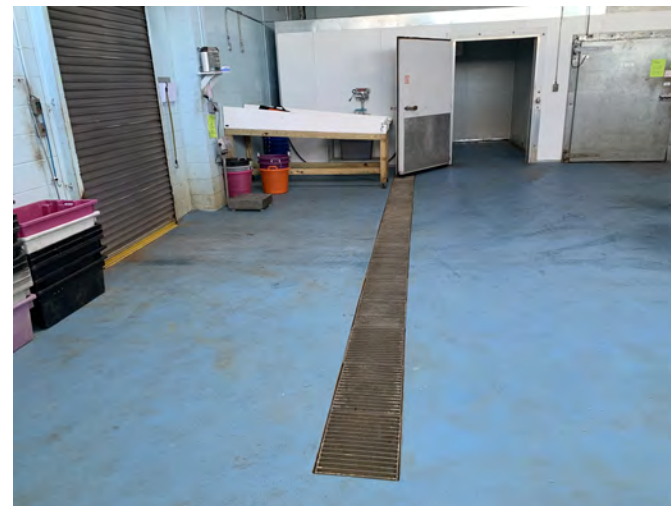
21. Floor drain trench observed in new addition building located north of Building 6.
