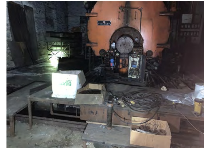
19. No. 6 oil boiler and trench filled with water located in Boiler Room where reportedly a small leak occurred.
