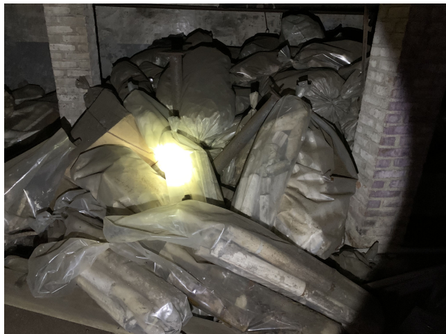
31. Numerous bags of asbestos containing pipe insulation observed in the basement of Building 1.
