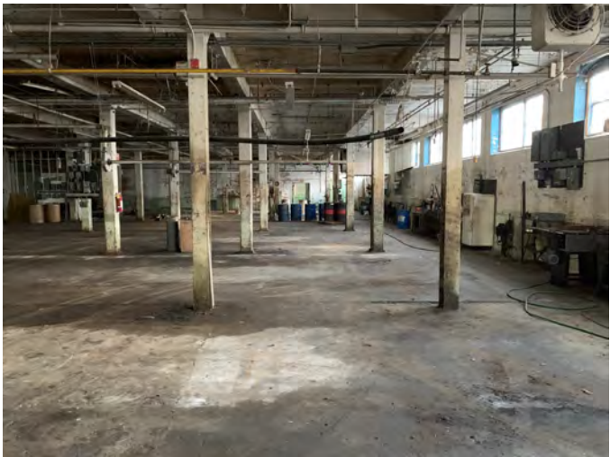
13. Staining observed on concrete floor in Building 7 & 7A.
