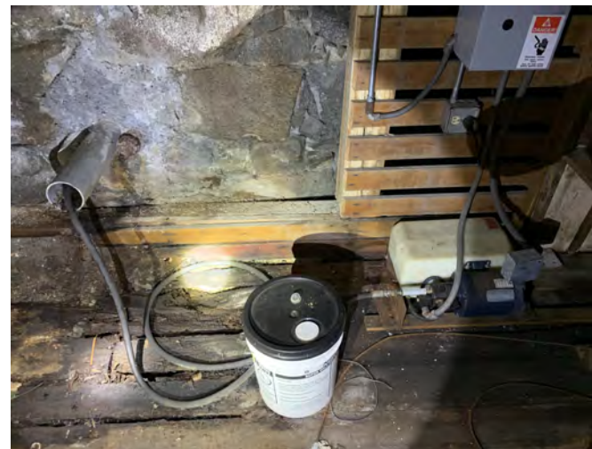
5. Oil reservoir for hydraulic lift and staining observed in basement of Building 1.
