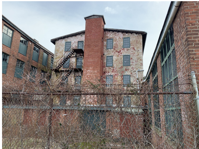
28. Possible lead-based paint observed on exterior wall on west side of Building 1.
