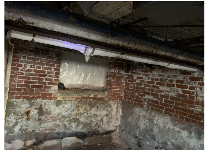
30. Possible asbestos containing pipe insulation observed in the basement of Building 3.
