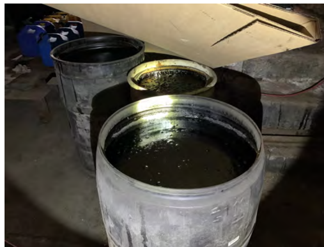
8. Drums containing 1 to 2 inches of No. 6 oil and water observed in the Boiler Room.
