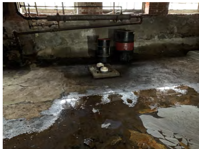
7. Oil observed on standing water located adjacent to leaking drums in the basement of Buildign 3.
