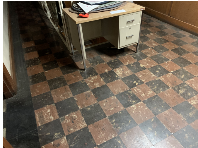
29. Possible asbestos containing floor tiles observed in office area located in Building 4.
