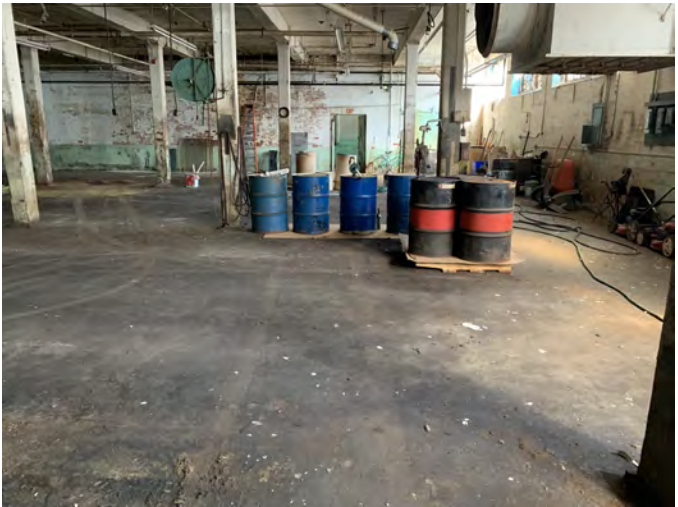
11. Drums containing lubricating oil stored in the basement of Building 7. Staining observed on the concrete floor.
