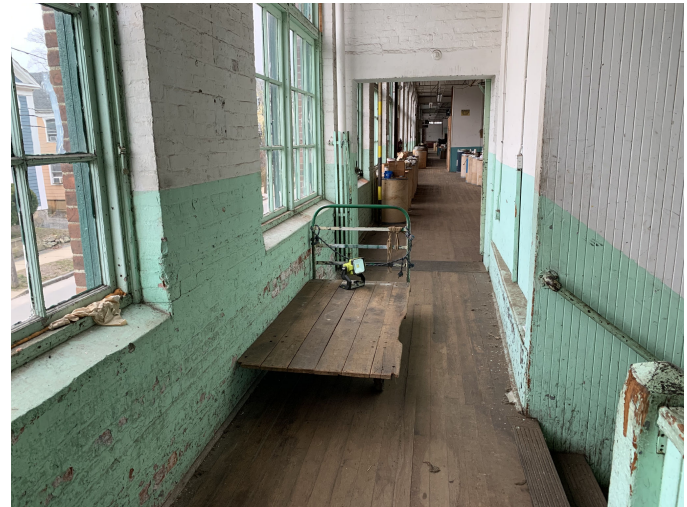
27. Possible lead-based paint observed on interior walls.
