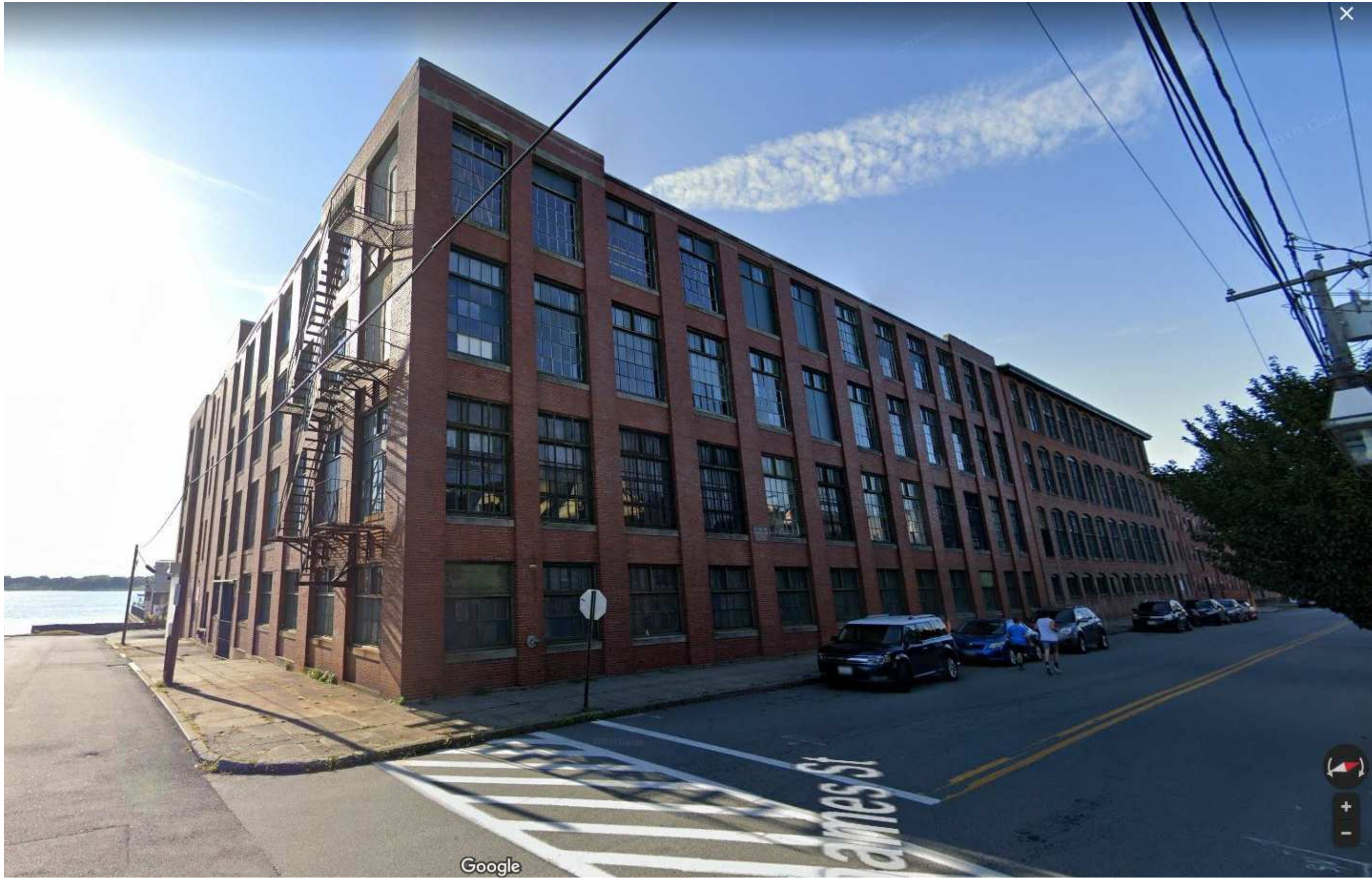
VIEW LOOKING WEST (BEFORE)
