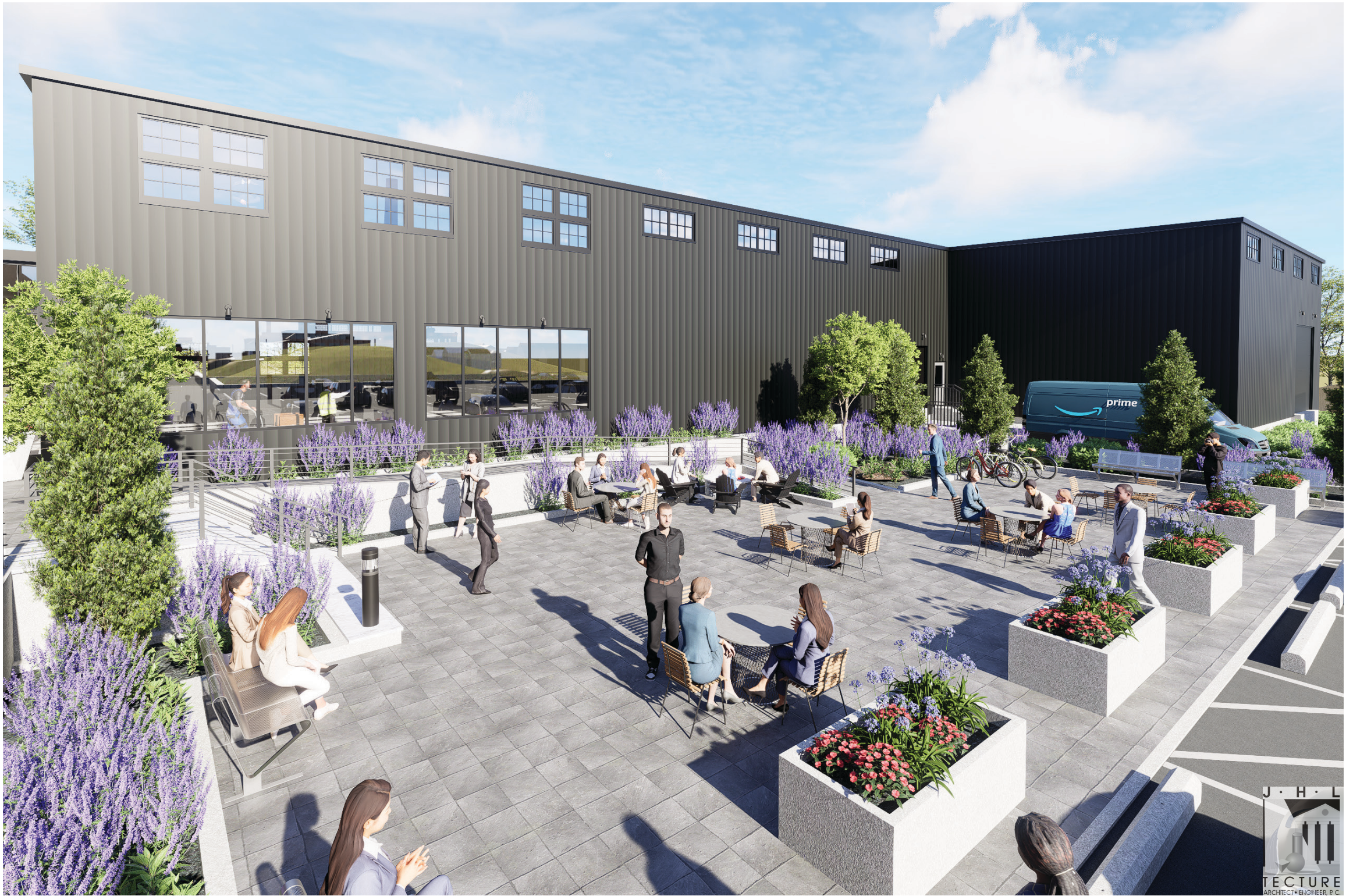
View 7: From entry courtyard, looking Southeast at new Unit 320 pre-engineered metal building
